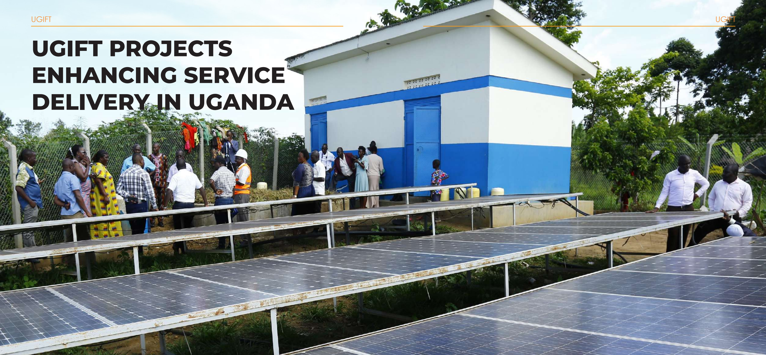
World Bank Team inspecting UGIFT supported irrigation system in Hoima
