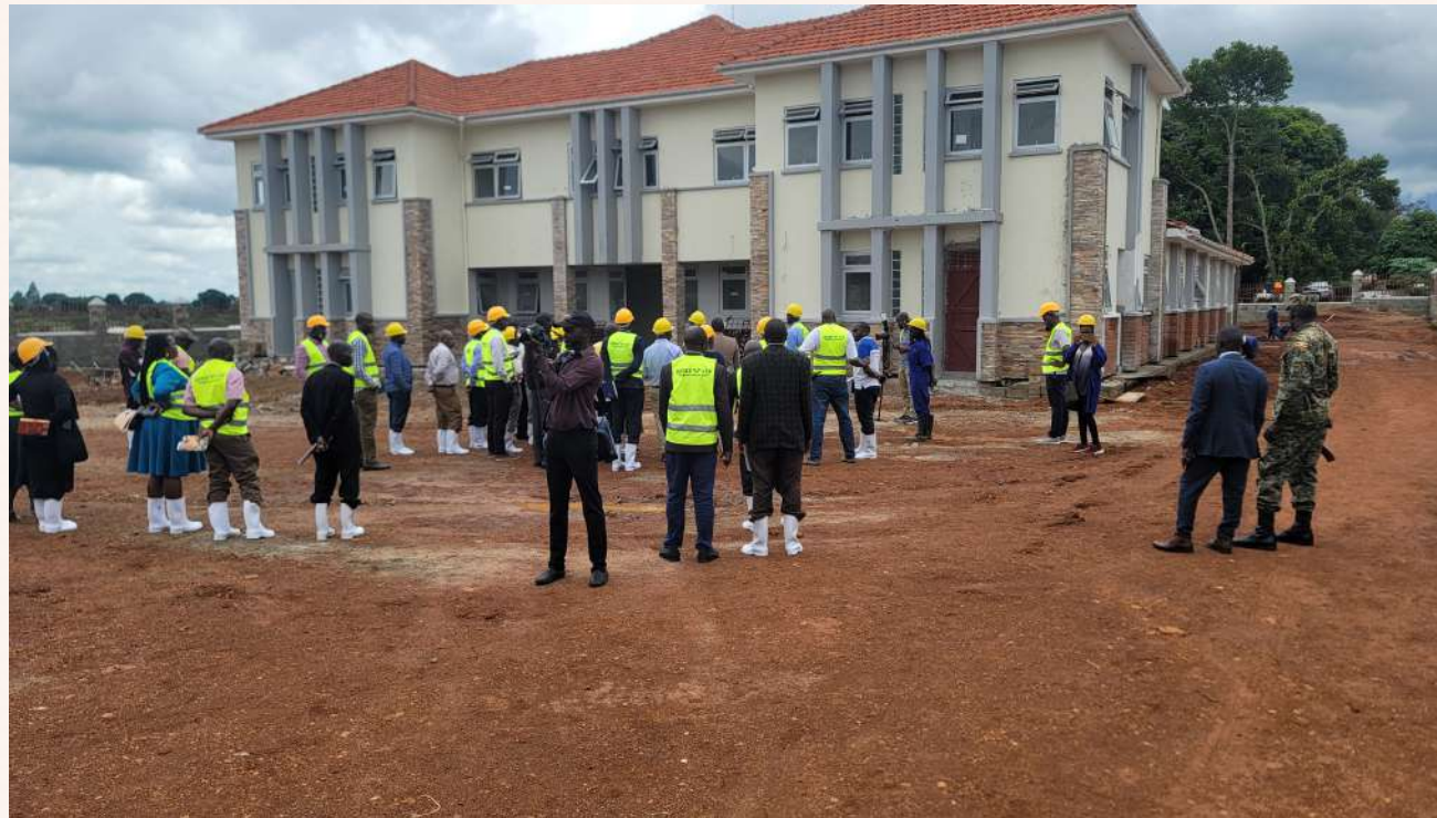
World Bank mission team inspecting completion works at Hoima blood bank recently.
