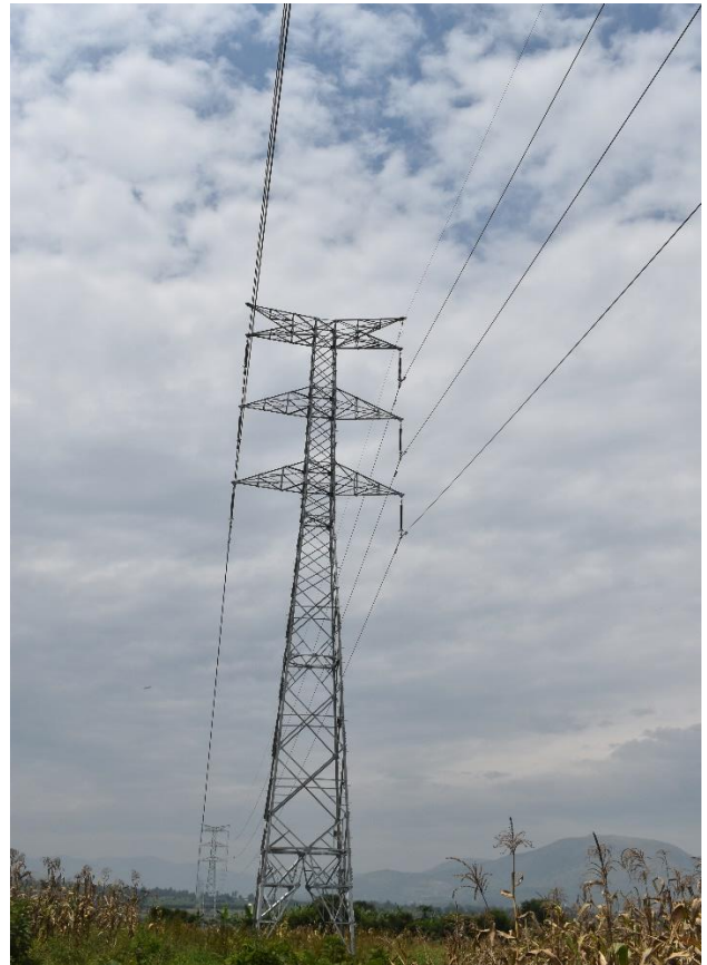
L-R: Completed resettlement house on the Kabale-Mirama Transmission Project; Part of a strung section on the Mirama-Kabale Transmission Project in Ntungamo District
