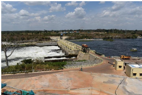
L-R: Completed spillway and dam structure; Inside the completed powerhouse building at Karuma HPP
