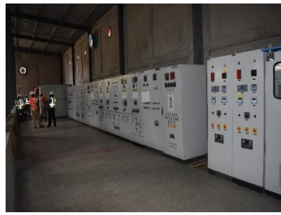
L-R: Completed dam structure at Nyagak III HPP; Newly installed control and switching panels in the Nyagak III powerhouse
