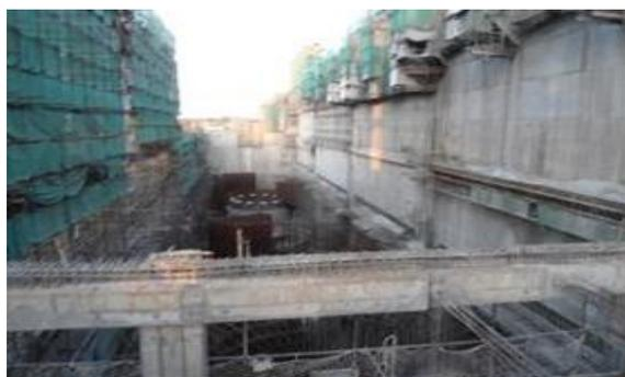
**Civil works for the generator foundations and installation of draft tubes and spiral casing in the powerhouse at Isimba HPP**
