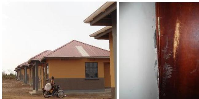
**L-R: Some completed units for the PAPs; Observed cracks near the door frame joint in one of the units in Kyakaboga, Hoima district**
