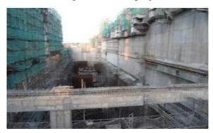
Civil works for the generator foundations and installation of draft tubes and spiral casing in the powerhouse at Isimba HPP
