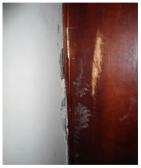
L-R: Some completed units for the PAPs; Observed cracks near the door frame joint in one of the units in Kyakaboga, Hoima district
