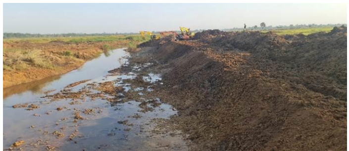
Dredging of River Tochi in Oyam District
