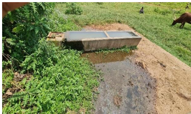
Kagango cattle trough depicting lack of maintenance
