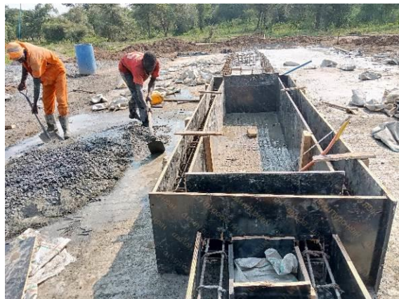
Reservoir tank tower for Mokoloyoro SSIS in Adjumani District; Cattle trough construction for Awal aboro SSIS in Gulu District
