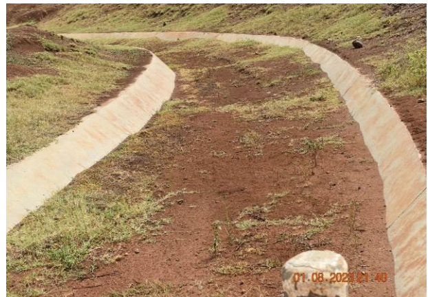
L-R: broken slabs were common in many parts of the scheme structures and silted auxiliary spillway at Ngenge river head works
