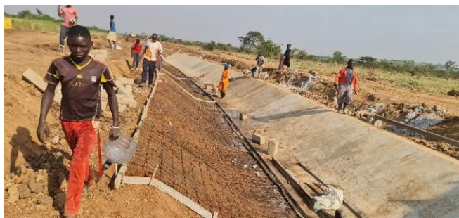
Casting a section of the main canal in Ragem, Packwach District
