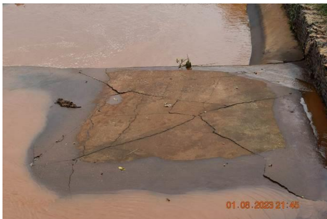
L-R: broken slabs were common in many parts of the scheme structures and silted auxiliary spillway at Ngenge river head works
