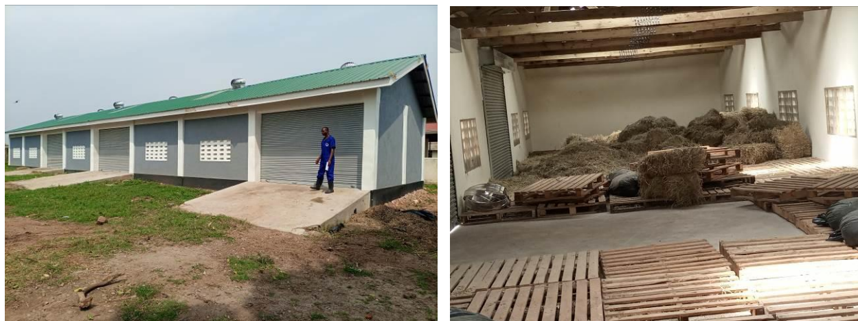
External view of the hay and storage facility (left) and internal view (right) that was constructed at LES in Wakiso District
