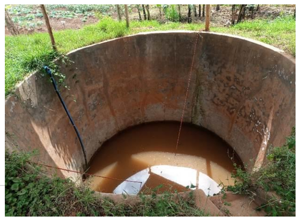
Horticulture crops garden with functional sprinkler irrigation (left) and improvised water source that had little water for irrigation as it was leaking (right)
