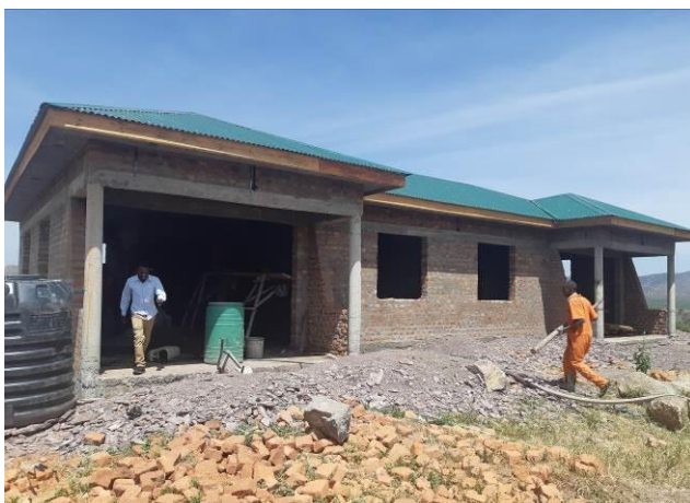
Junior staff quarters under construction at Maruzi in Apac District
