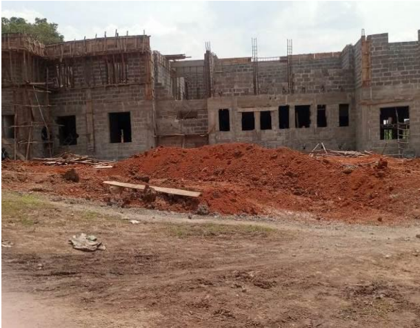
NARO administration building under construction in Namaleere Village Wakiso District
