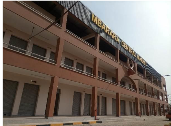
Construction of Mbarara Central Market in Muti Cell, South Division, Mbarara City was completed and facility was ready for use
