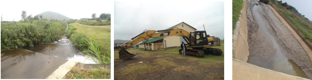
Left to Right: Diversion point from Mubuku I main silted channel and faulty excavator in Kasese District and silted main canal at Doho II Irrigation Scheme in Butaleja District
