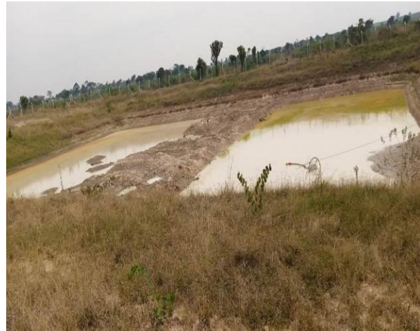
L-R: A silted valley tank of Kataigwa Scheme in Nabuganyi Parish, Kayunga District
