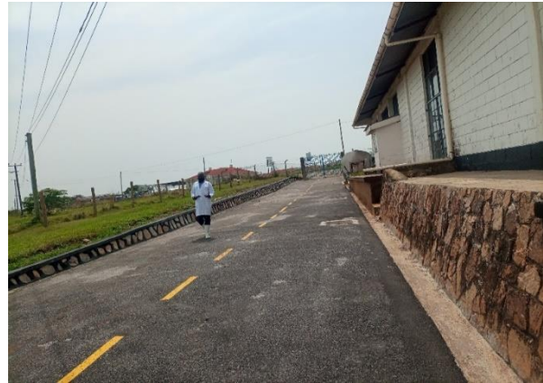
Completed access road to serve Entebbe Dairy Training School and Factory in Entebbe Municipality in Wakiso District
