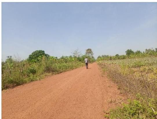
Completed community access road in Mataba Village, Kayunga District under a MAAIF project
