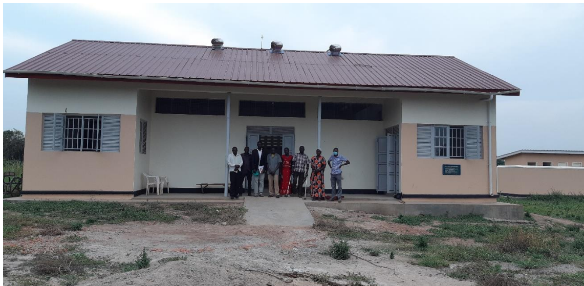
Substantially completed value addition facility of Atiira Farmers' Cooperative Society in Serere District
