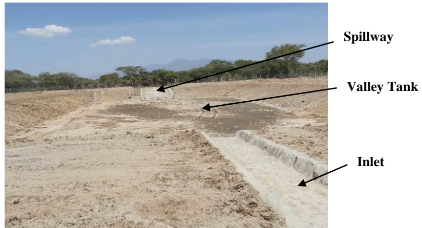
Arengetekai Valley Tank in Nabilatuk Sub-county, Moroto District
