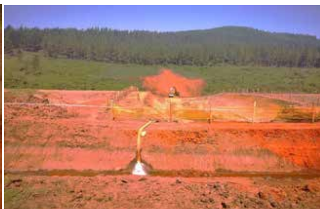
The diverted Mishumbi River and core trench excavations at Kabuyanda dam in Isingiro
