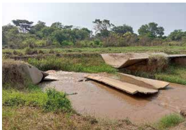
A section of a broken main canal of Wadelai Irrigation Scheme in Packwach district
