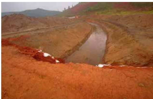
The diverted Mishumbi River and core trench excavations at Kabuyanda dam in Isingiro
