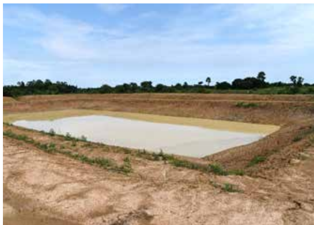
L: Excavation works for Onekogwok Valley Tank in Omoro district; R: Completed excavation for Oriyamai Valley Tank in Amolator Town Council, Amolator district
