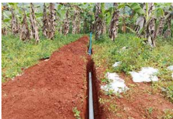
A distribution pipe laid for Namaitu medium scale irrigation scheme in Bududa district
