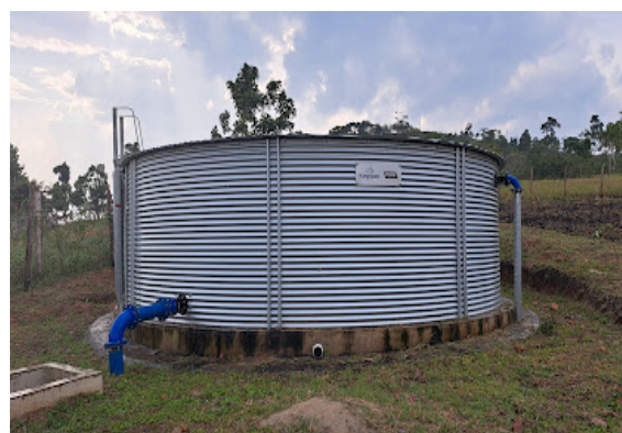
100m 3 reservoir tank for Kirema medium irrigation scheme
