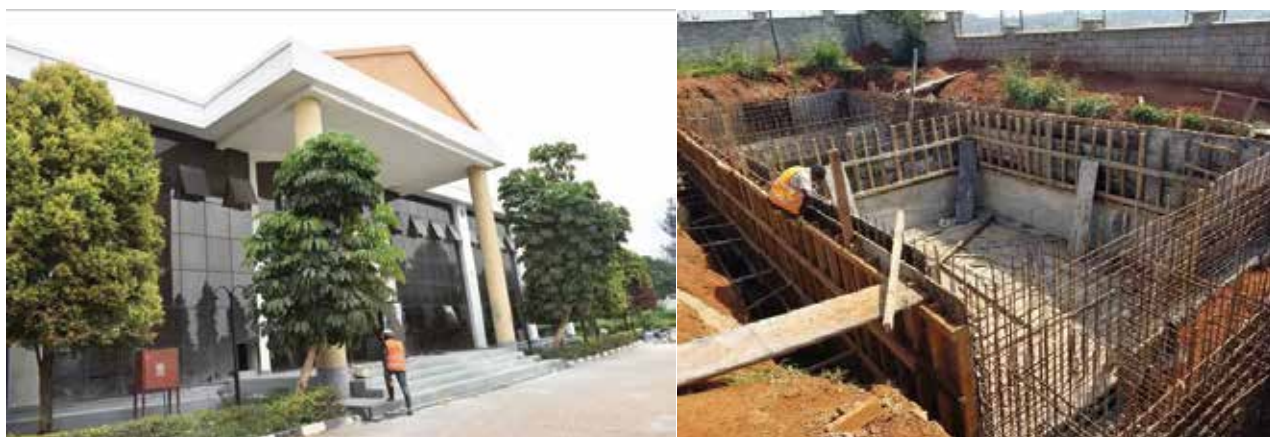
L-R: Rehabilitated Cassava Centre of Excellence structure at NaCRRRI; and effluent treatment plant under construction at the Anti-Tick Vaccine Facility in Wakiso District
