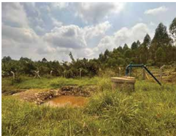
Intake at Nadangira Small-Scale Irrigation (SSI) Scheme in Nadangira Village, Kakiri Town Council, in Wakiso District
