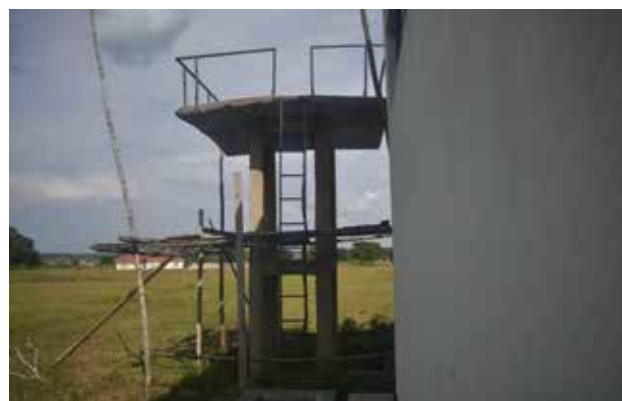
L-R: Completed Milk Collection Centre in Bukedea Town Council; and complete tank stand with a warped slab at the same facility
