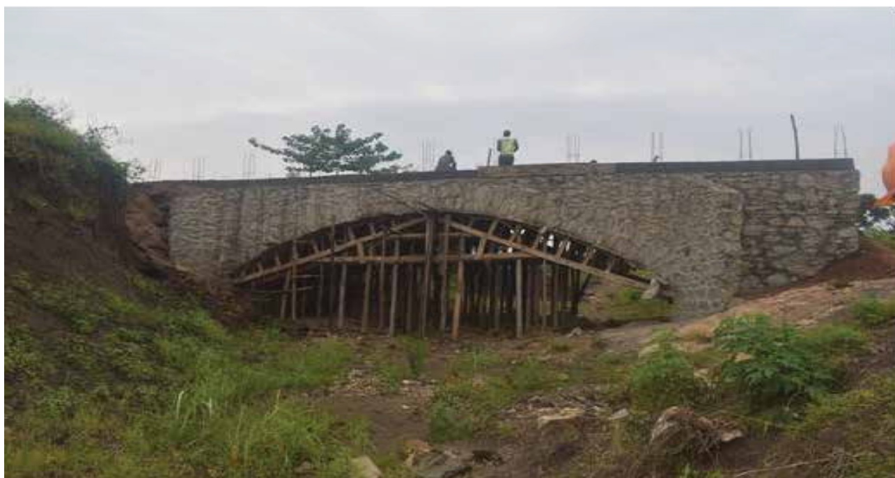
Ongoing works for a road choke (bridge) at Nansasa Village, Bunghobi Sub-county, Mbale District funded by NOSP
