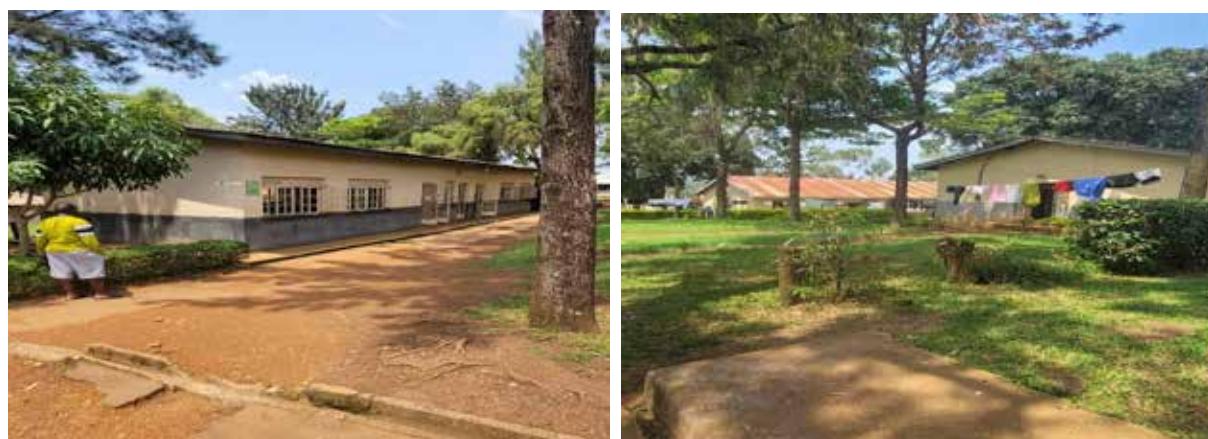
L-R: Formerly Bunyoro Rural Training Centre, now housing Hoima Nursing and Midwifery Institute
