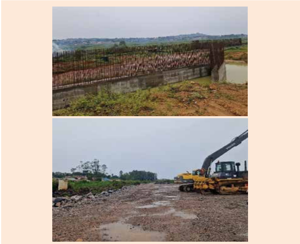
Figure 8: Photo Montage of Construction Works at the Busega-Mpigi project
