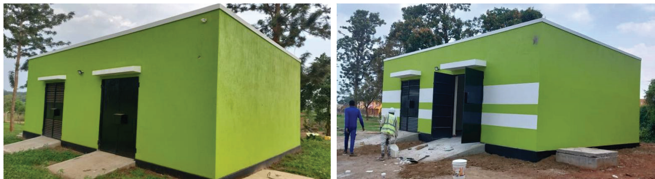
L-R: A completed structure to house the transmission site at Kayunga District headquarters. A nearly completed structure to house a transmission site at Iganga under the GOVNET-PHASE V Project.
