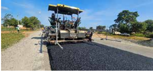
Ongoing Paving along the Soroti – Lira road section
