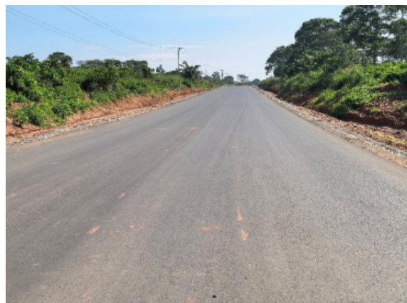
Luweero-Butalangu: Completed asphalt layer at Km 21+500 in Nakaseke district
