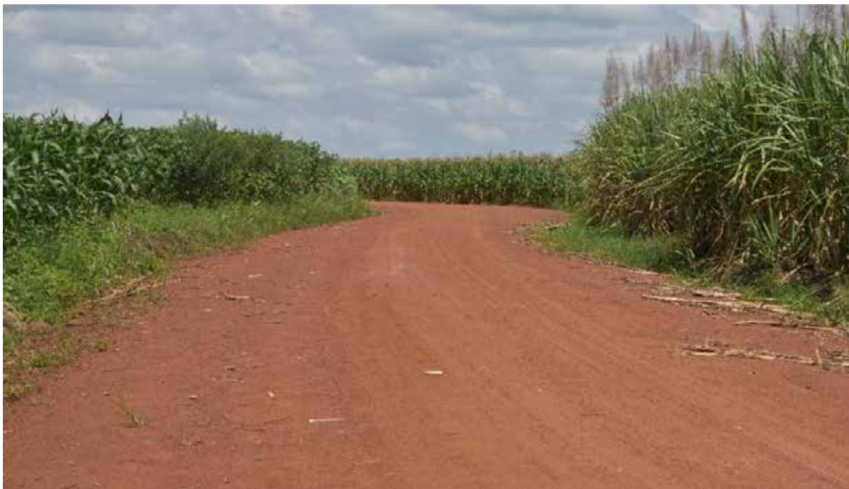
Rehabilitated 2.8Km Kiruli-Kisasa Road in Kiruli Subcounty, Masindi District.
