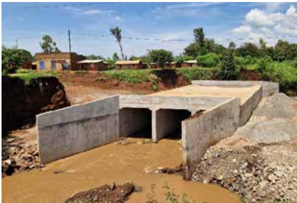
Muyembe-Nakapiripriti: Completed three-cell Box culvert at km 55+240
