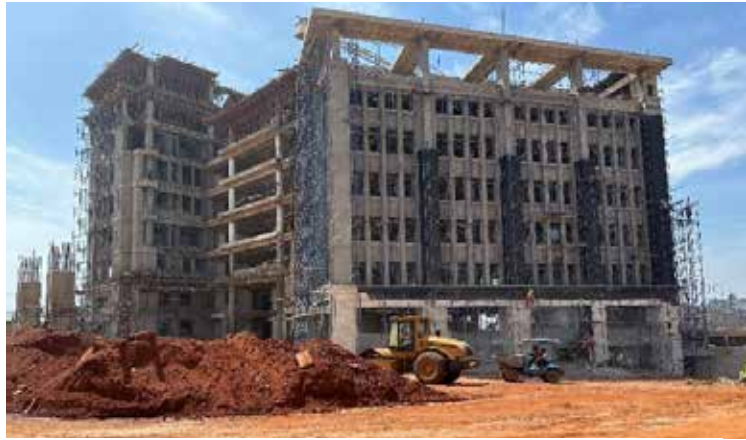
Construction of the Skills Development Headquarters at 55% at Kyambogo
