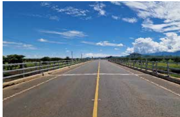
Completed section of Muyembe-Nakapiripriti at km 42 + 230
