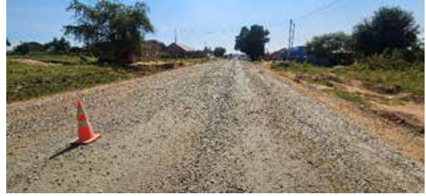
Yet to be processed base layer along the Soroti – Lira section
