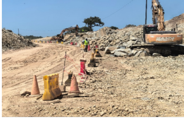
Koboko-Yumbe-Moyo: Ongoing rock excavation at Km 97+200 in Moyo district
