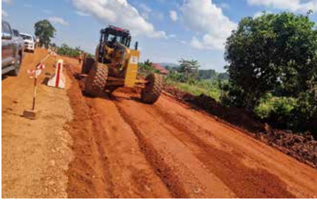
(Kihura)-Bwizi-Rwamwanja-Kahungye/Mpara-Bwizi Road Project, L-R: Preparation of fill layers at km 2+400; Asphalt concrete Plant Assembled at the Contractor's Camp in Preparation for asphalt Works
