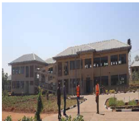
Completed Administration Block at Amelo Technical Institute in Adjuman District.
