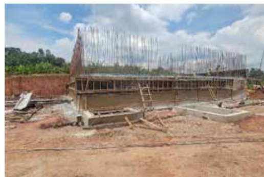
Construction ongoing at Nyabushenyi Sump at Isingiro WSS in Isingiro District
