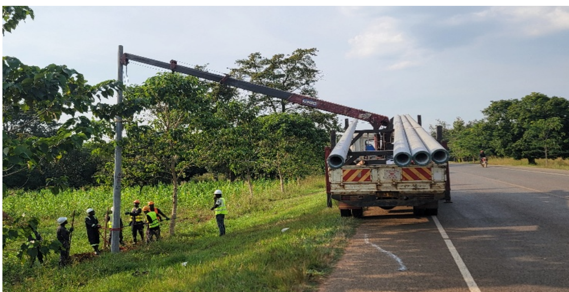
Pole erection along Gulu-Kitgum road
