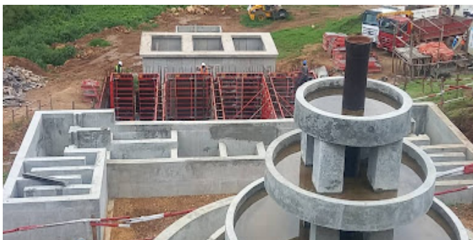
Bitsya treatment plant (raw water abstraction tank, coagulation, sedimentation, filtration and clear water tanks)
