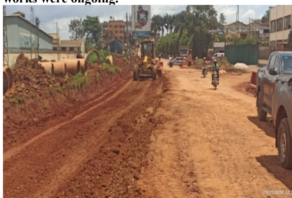
A section of Eighth Street in Makindye Division under Lot 3 at Km 0+300 where sub0-base works were ongoing.
