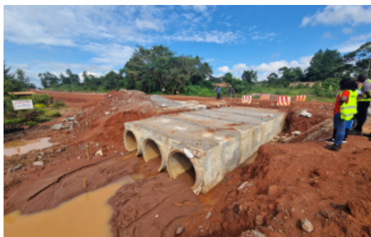
Three cell pipe culverts under construction on Luwero-Butalangu Road.
