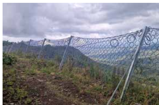
Rock fall fencing barrier installed to protect Kapchorwa-Suam Road.
