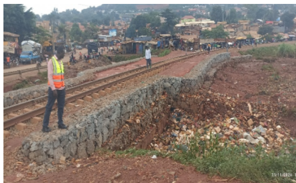
The Kinawataka drainage gabion protection works.
