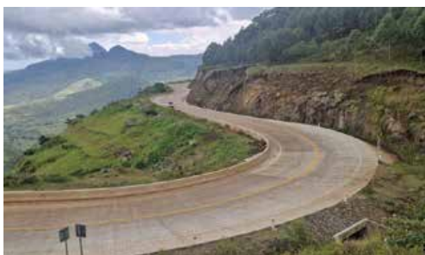
A completed section of a rigid pavement along Kapchorwa-Suam Road.
