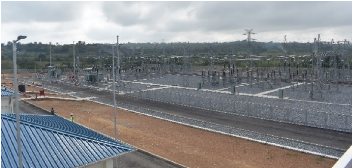
Completed switchyard at the new 132 kV Agago substation.
