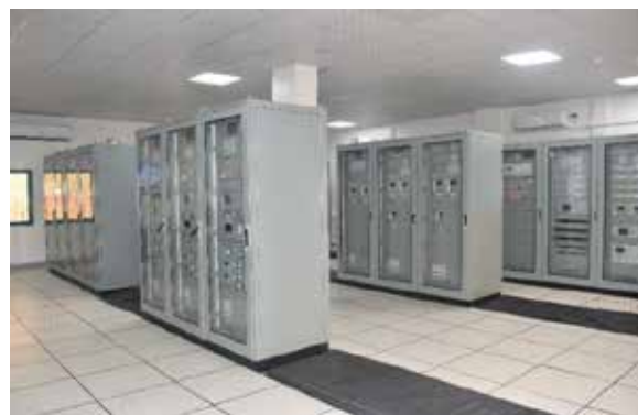
L-R: Completed substation plant house; commissioned control/protection panels at the Agago 132 kV substation switchyard.
