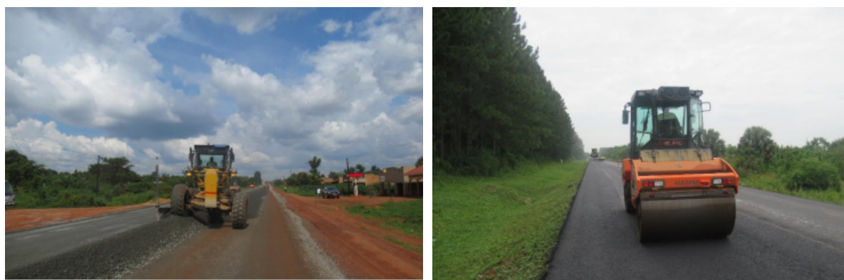
Base works ongoing along the Lira-Kamdini section. Asphalt works along the Dokolo-Lira section.
