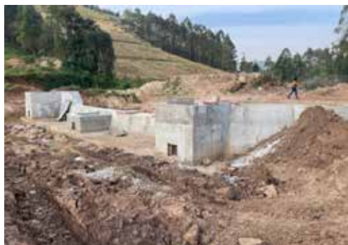
Bitsya treatment plant (raw water abstraction tank, coagulation, sedimentation, filtration and clear water tanks)
