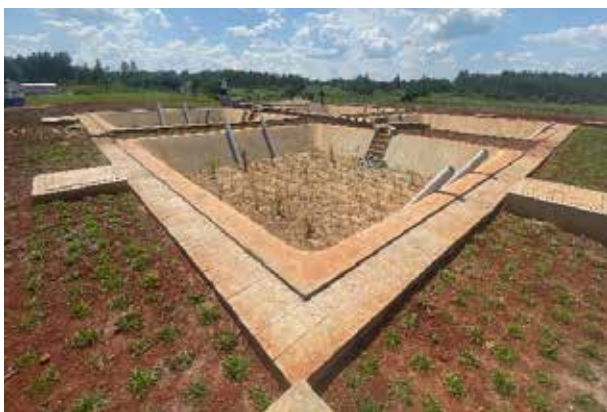
L: Planted drying beds for Busia FSTF; R: Sludge ponds for Koboko FSTF
