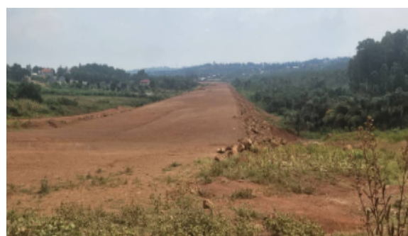
Completed fills in the swampy sections along the road.
