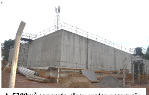
A 5200m 3 concrete clear water reservoir at custom corner in Gulu district
