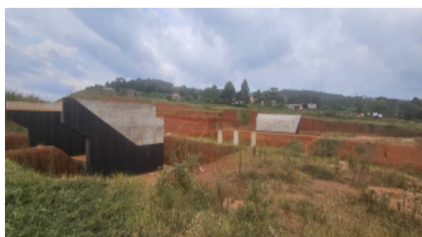
Completed abutments for one of the bridge structures.
