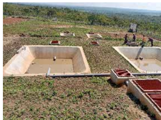
L: Planted drying beds for Busia FSTF; R: Sludge ponds for Koboko FSTF
