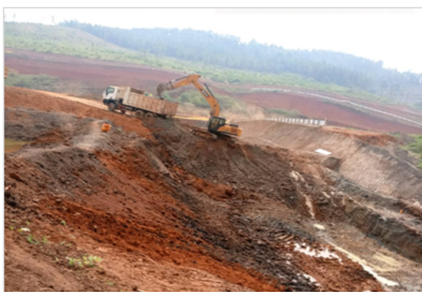
The intake excavation works and diverted Mishumbi River at Kabuyanda Dam in Isingiro
