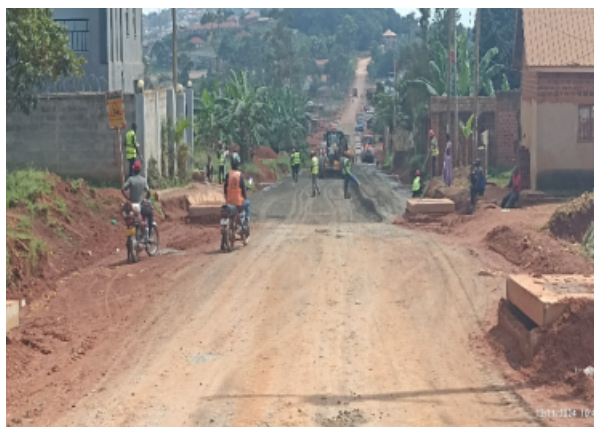
A section of Mugema Road in Rubaga Division under Lot 5 at Km 1+800 where placement of CRR works were ongoing.
