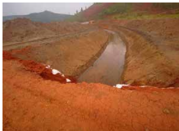
The intake excavation works and diverted Mishumbi River at Kabuyanda Dam in Isingiro
