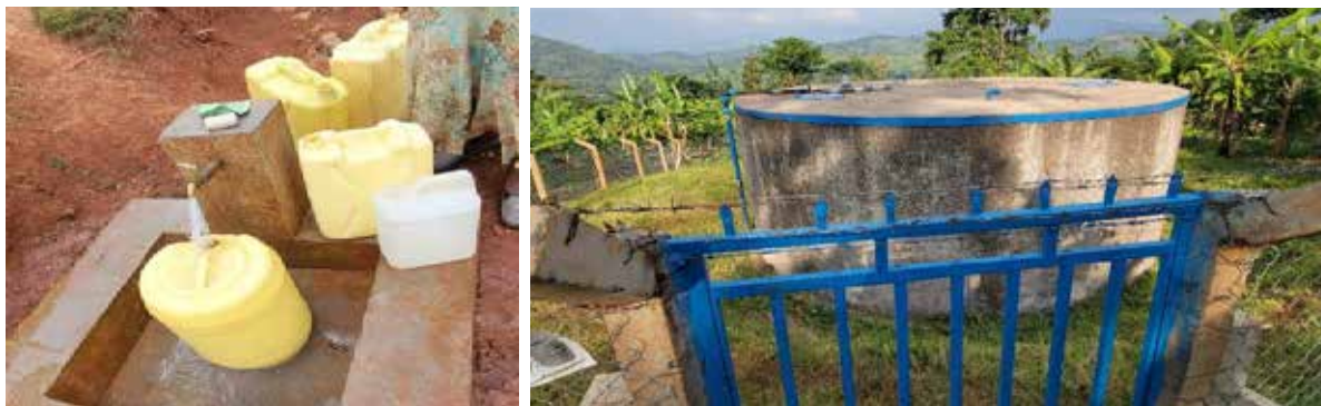
L-R: A tap stand at Atar Village, Kirwoko Parish, Kween District; a reinforced concrete water tank at Bumakusa Upper Village, Ikaali Parish, Manafwa District.
