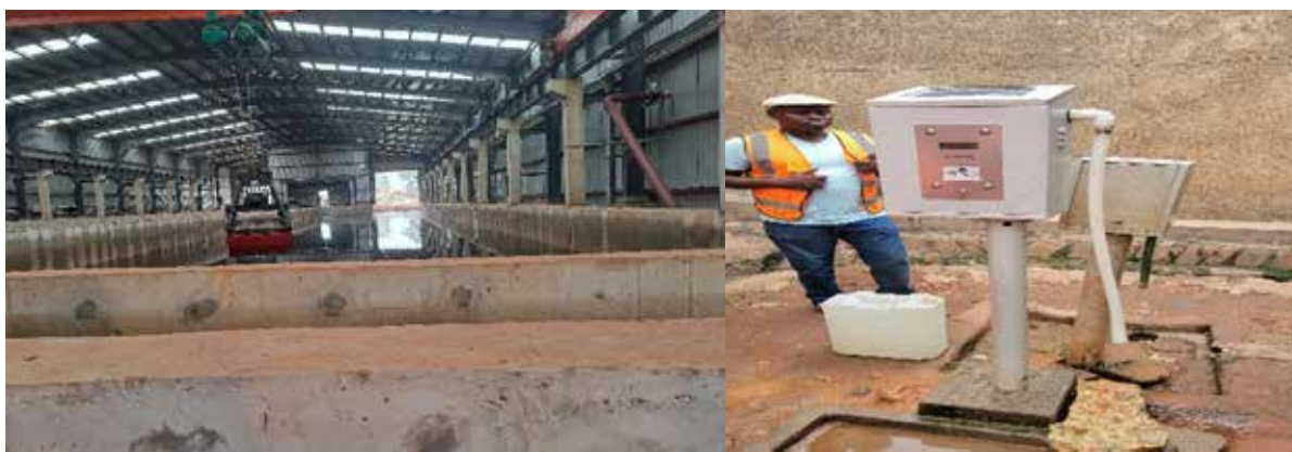
L-R: Constructed sedimentation tank at Nalukolongo faecal treatment plant; prepaid meter installation in Mulago informal settlement.
