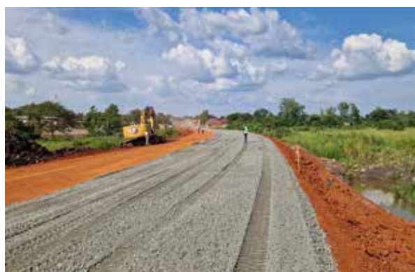
Construction of base layer along Rwenkunya-Apac Road.
