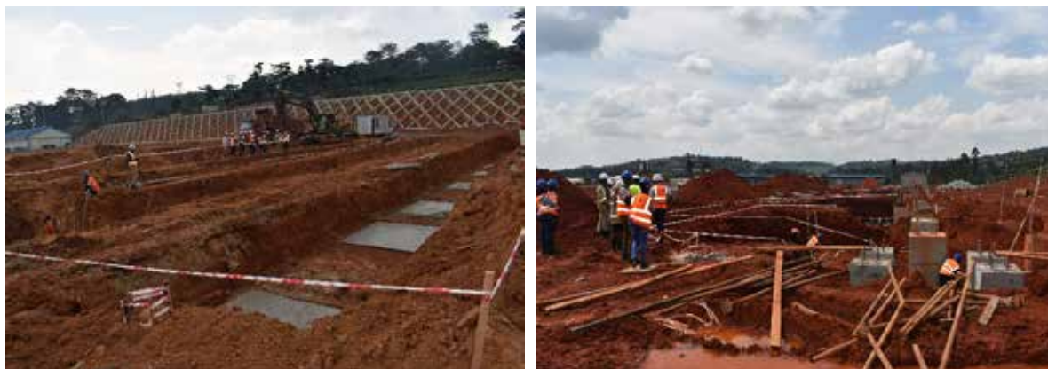
L-R: Excavation of equipment foundations at Mukono substation; completed equipment foundations and ongoing excavations at Buloba substation.
