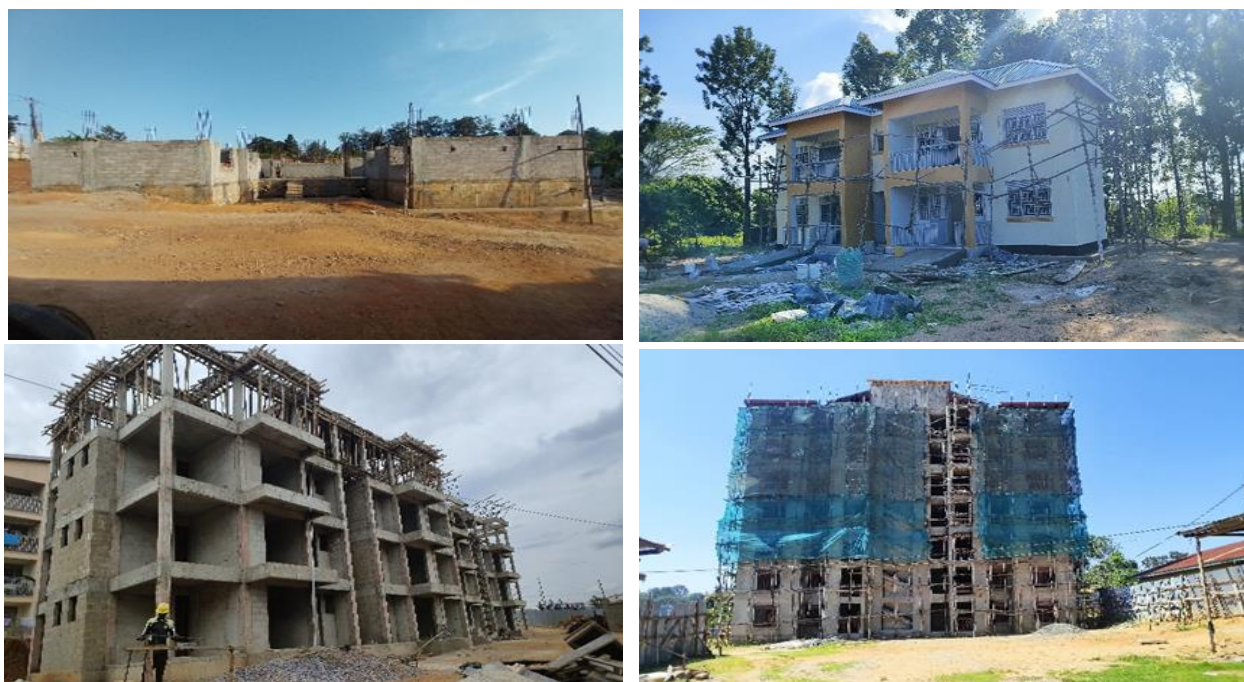
Clockwise: Masaka, Vurra Port, Arua and Mbarara health workers' accommodation blocks
