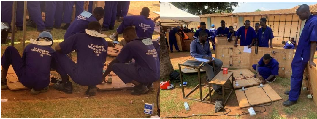
L-R: Some of the 123 students doing UBTEB practical electrical installation exams: A student presenting his UBTEB electrical installation work to the Assessor at St. Joseph's Technical Institute-Kisubi
