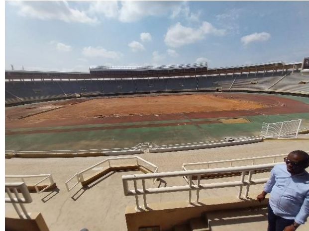
Status of ongoing renovation of the pitch at Namboole Stadium
