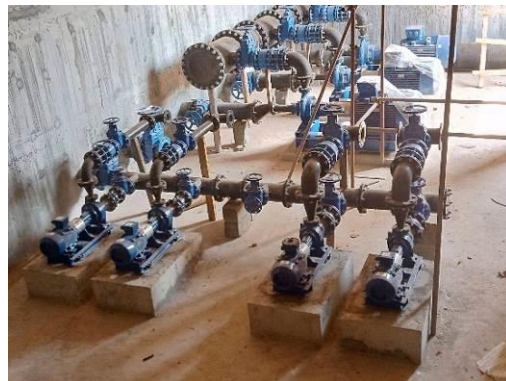
L-R: Pipe laying of the Karuma-Gulu Transmission Mains; Installed uplift pumps of Karuma Water Treatment Plant in Nwoya District
