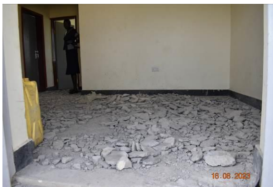
L-R: Failed floor hacked for rehabilitation at Priscilla Girls Comprehensive Secondary School in Katakwi District
