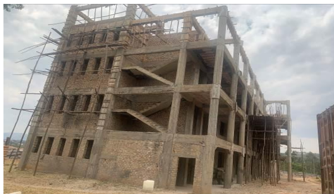
Construction of the Science Laboratory Block at Bishop Stuart University-Mbarara
