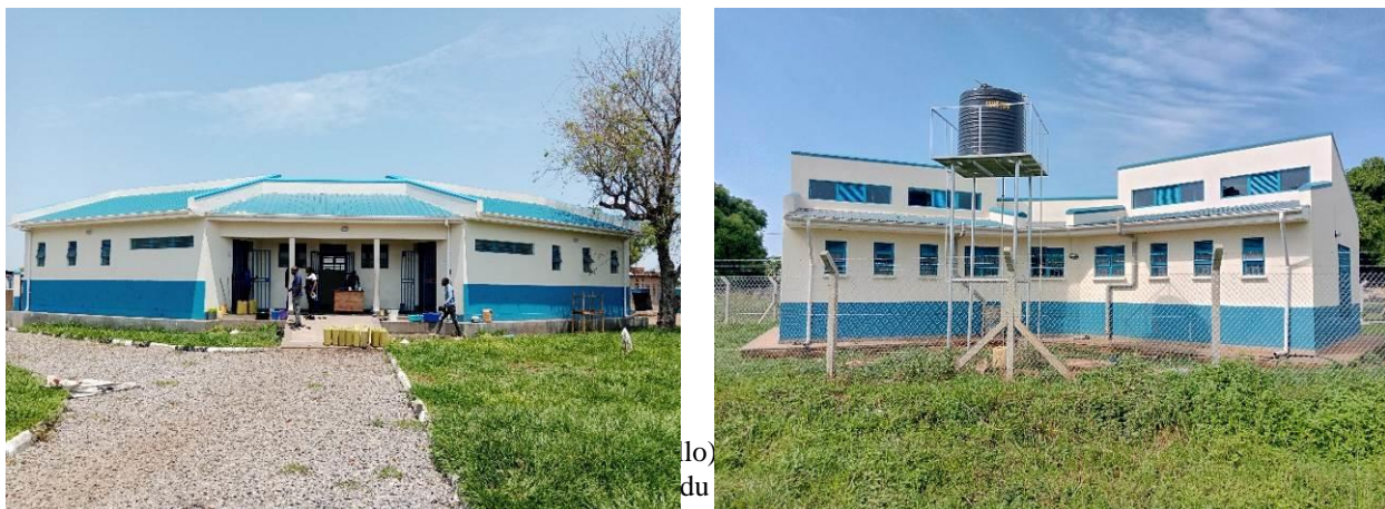
L-R: Public sanitation facilities of Bubia-Elegu WSS; and Atiak WSS in Amuru District
