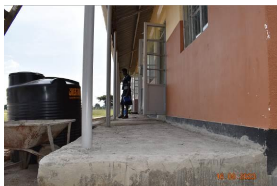
L-R: Failed floor hacked for rehabilitation at Priscilla Girls Comprehensive Secondary School in Katakwi District
