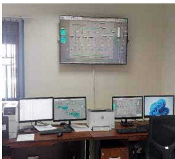
L-R: A prepaid PSP and installed a Supervisory Control and Data Acquisition (SCADA) system control unit.
