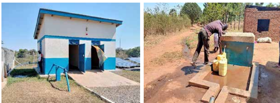
L-R: A pump/guard house, and a PSP for Adwong solar-powered WSS in Alebtong Town Council.
