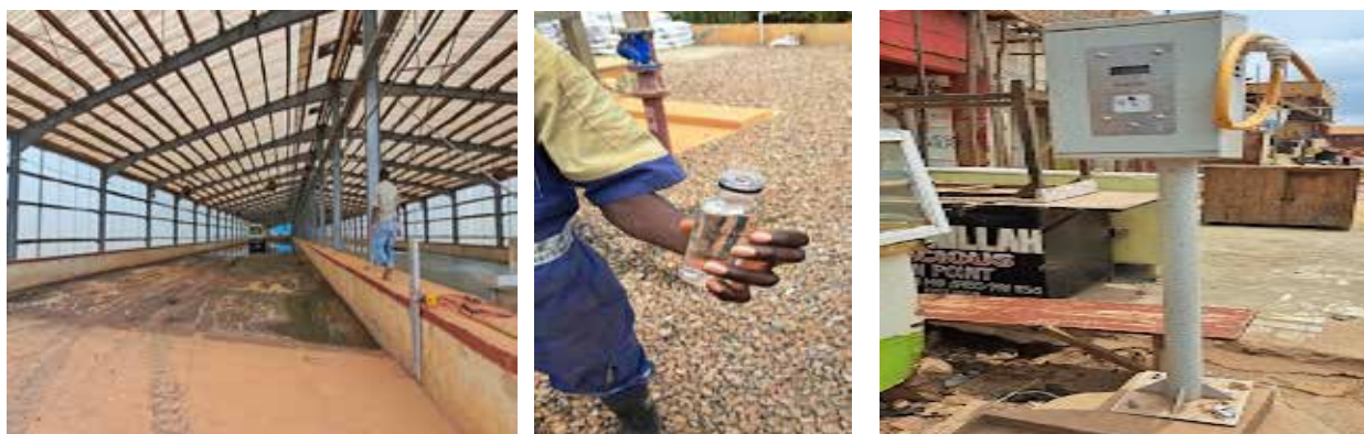
L: A section of the sludge drying bed; C: Final treated sewage water that is discharged into the wetland from Nalukolongo FSTF in Wakiso District; and R: A prepaid water meter in Nalukolongo
