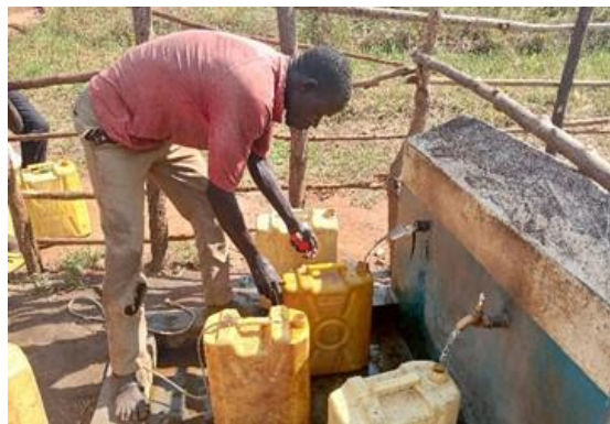
L: A public stand post (PSP) with broken tap; R: Two 10m 3 reservoir tanks for Ogwari WSS in Lakalac Parish, Nwoya District.
