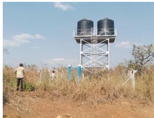
L: A public stand post (PSP) with broken tap; R: Two 10m 3 reservoir tanks for Ogwari WSS in Lakalac Parish, Nwoya District.
