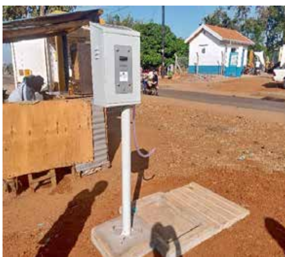
L-R: A prepaid PSP and installed a Supervisory Control and Data Acquisition (SCADA) system control unit.
