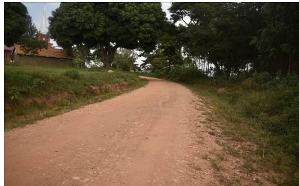
One of the opened, graded and graveled roads in Ndejje University, done in preparation for the hosting of the East African University games in December 2022
