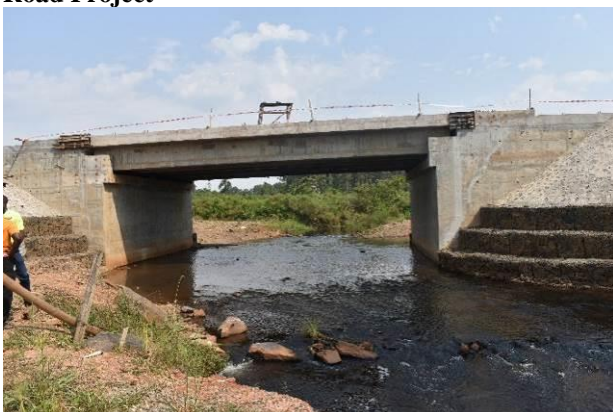
Completed Fjumangabo bridge at Kms 17+163 along the Kabaale-Kiziranfumbi (25kms) Road Project on Oil Road Package 5
