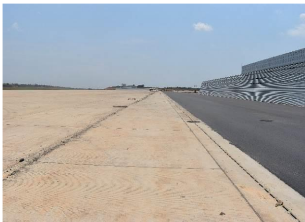
Kabaale International Airport: The parking apron in front of the terminal building
