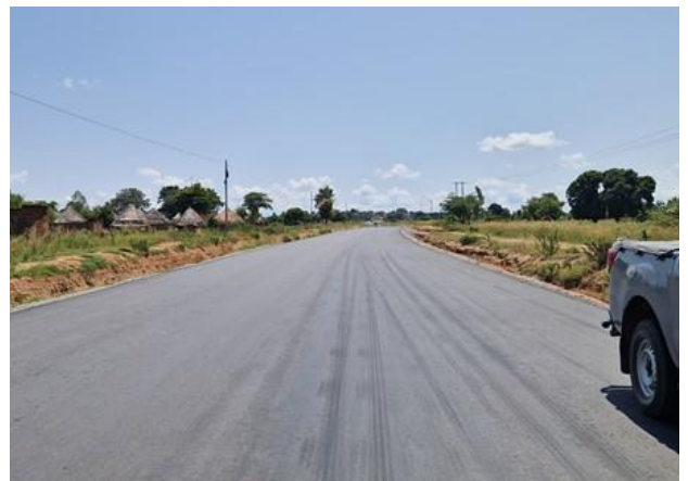
Tarmacked section of Alwii-Nebbi Road, port of the priority section
