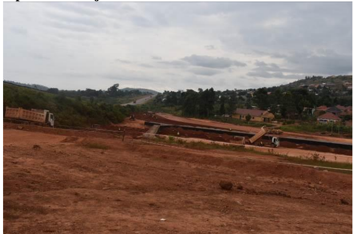
Bridge construction at interchange No.3 (kms 12+500) on the Busega-Mpigi Expressway Road
