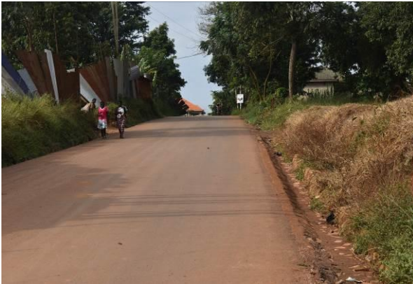
Blaire Road in Kira Municipality paved with asphalt pending road marking
