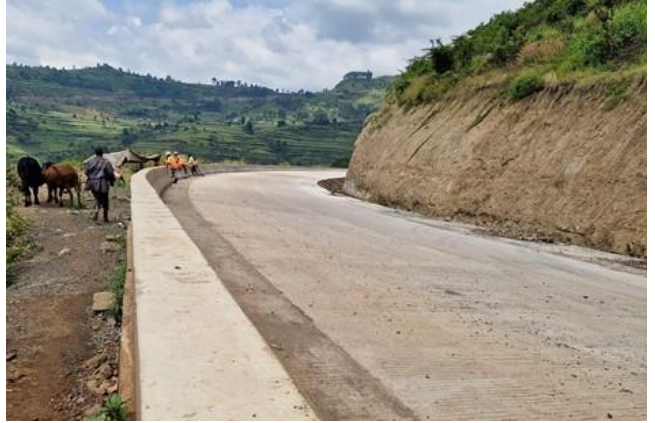
Completed section of rigid pavement along Kapchorwa- Swam Road Project
