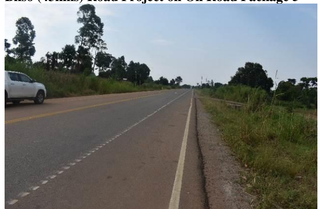
A completed section at Kms 19+000 along the Hohwa-Nyairongo-Kyarushesha Road Project on Oil Road Package 5
