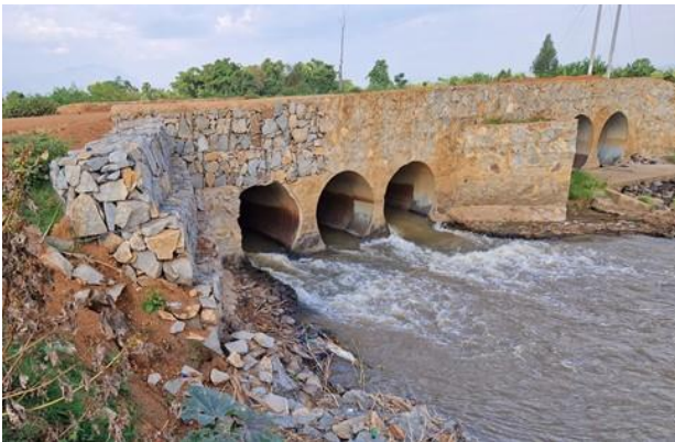
Tororo UNRA Station: Emergency works on Kachonga-Kidoko-Magodes Road
