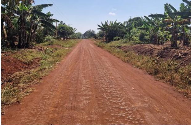
Bugiri District: A section of Muterere-Kimbale after routine mechanized maintenance
