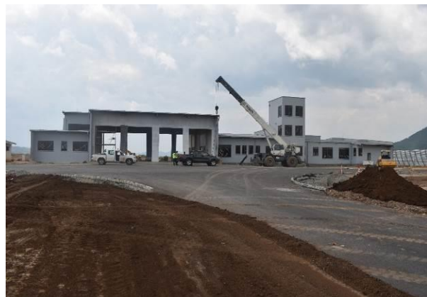
Kabaale International Airport: The Rescue and Fire Fighting Facility under construction
