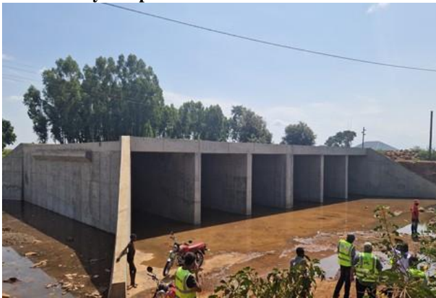
Six cell box culverts constructed along Muyembe-Nakapiripiriti Road
