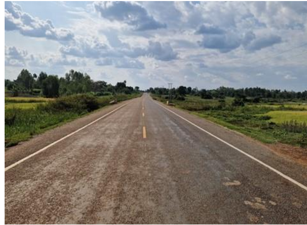
Tororo UNRA Station: Nagongera–Busolwe–Busaba after (kms) was upgraded from Gravel to Bituminous Low Volume Seal Road
