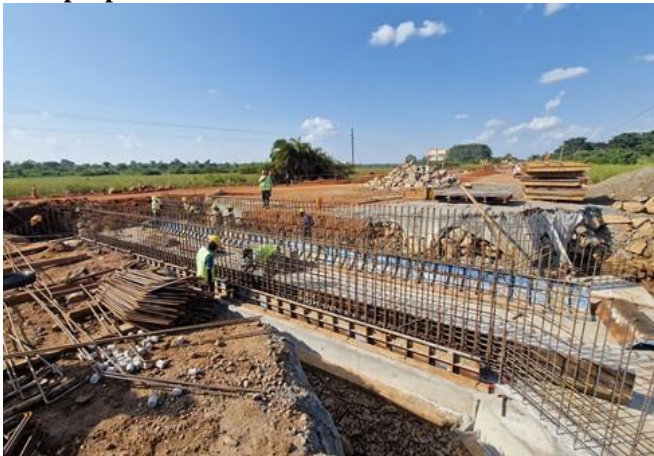
Construction of a box culvert along the Apac-Lira Road section
