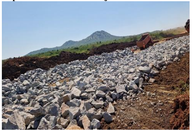
Rockfilling of a swamp section along the Rwenkuny-Apac Road Project
