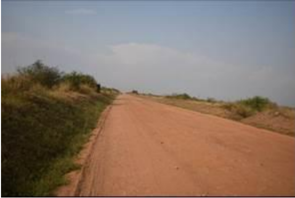
Kasese UNRA Station: A well-graded and shaped section of L.Rwentare-L.George Road at the start (kms 0+000)
