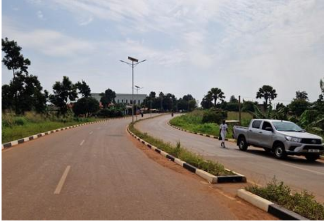
Gulu Logistics Hub Access Road – the project was substantially complete
