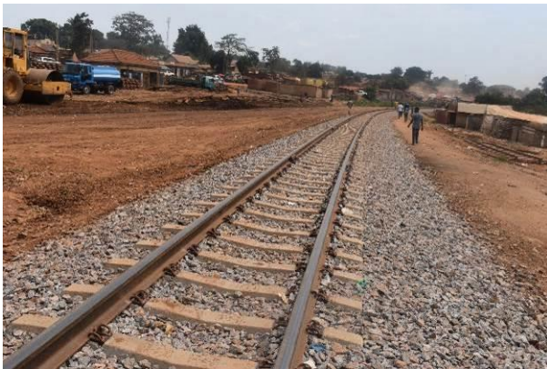
A completed section of the railway line at Namanve Station
