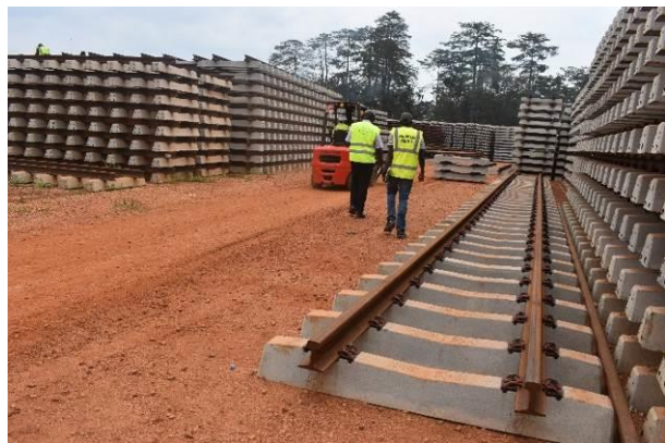
Assembled rail tracks at the Kawolo-Lugazi
