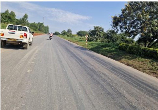
Rehabilitated section of Lira – Kamudini Road section
