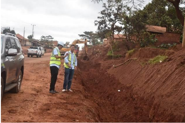
Excavation works for the roadside drain at Ggangu along the Munyonyo Spur on the Najjankumbi-Busabala Road Project
