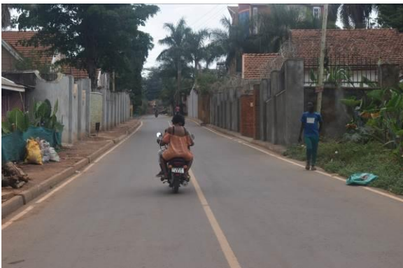
A marked Katuramu Lane in Bukasa – Makindye Division pending completion of paving the walkways
