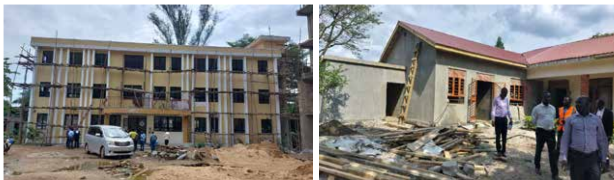
L-R: A substantially complete GMP facility at the Natural Products Research & Innovation Centre - Busitema University Mbale Campus. Construction of Laboratories for space science and lithium battery projects at Busitema University Nagongera Campus
