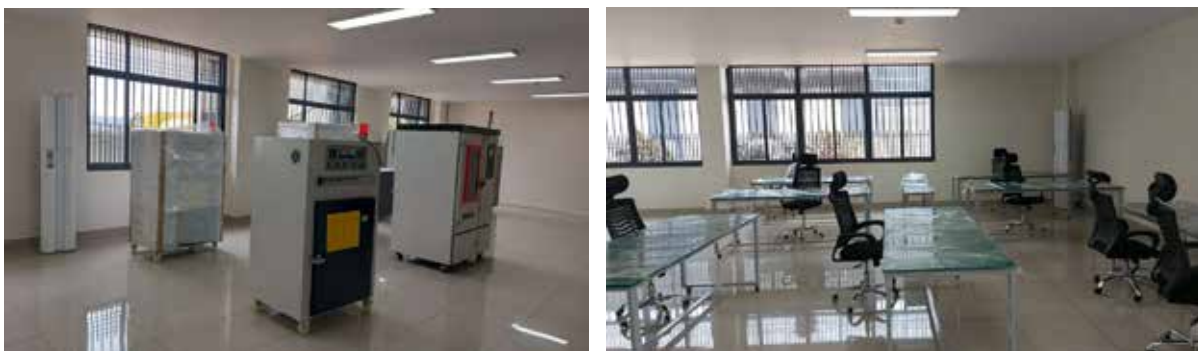
L-R: Installed equipment, and Workstations at Lwera Electronics workspace at TIBIC-Namanve
