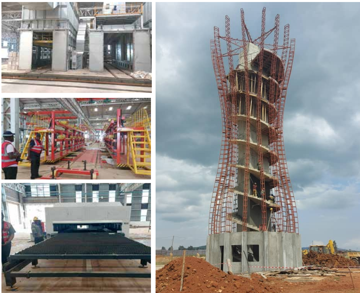
Top left to left bottom: Paint shops nearing completion, Installed bus assembly stations, High density Computer Numerical Control machine. Left: Watch and communication tower under construction at Kiira Motors Plant in Jinja District
