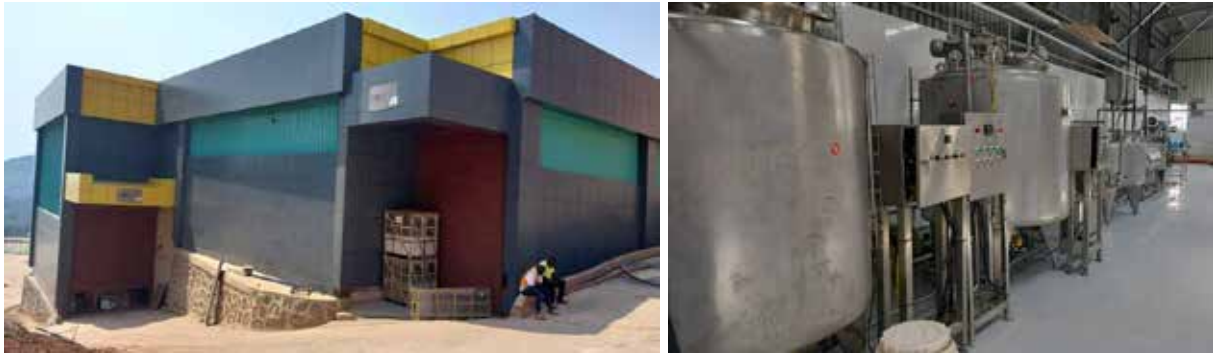
L-R: A substantially complete 100 MT warehouse and a ready-to-drink coffee production line at Inspire Africa coffee factory at Rwashamire, Ntungamo District
