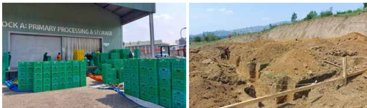
L-R: Stacked tray of green bananas awaiting peeling and processing at Nyaruzinga-Bushenyi District. Foundation works for the Shuuku collection centre in Sheema District
