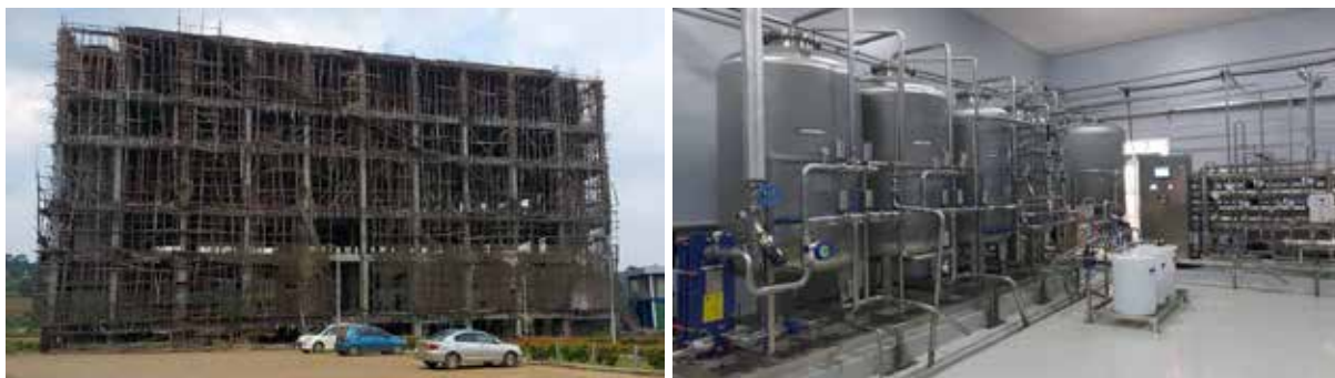
L-R: Hormone facility under construction at Dei BioPharma in Matugga. A purified water treatment system at Dei BioPharma in Matugga, Wakiso District
