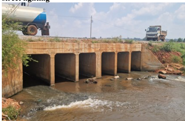
Kiwologoma-Kitukutwe-Kijabijo Road in Kira Municipality: Six-cell box culvert constructed across Lwajjali Wetland
