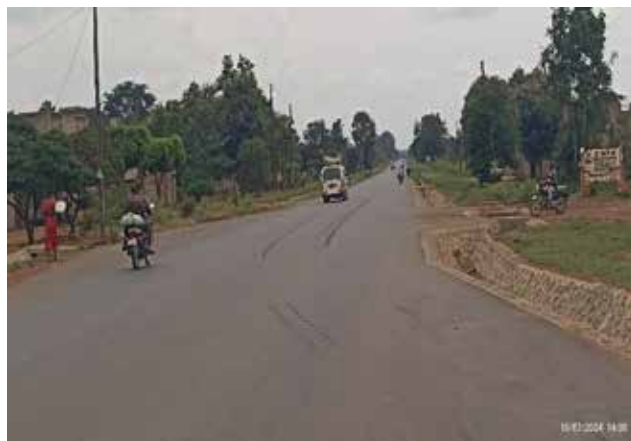
Lot 2B Lira-Kamdini section: Completed road section with asphalt pavement and stone pitch-lined side drains at Km 137+720
