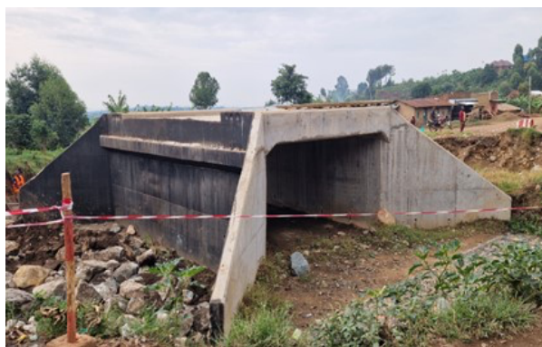
Box Culvert at Nyabuswa along Bukuku – Rubona in Kabarole District, awaiting backfilling
