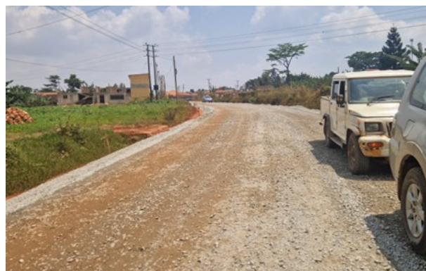
Construction of the base layer along Bulindo-Nsasa-Namugongo road (4.56km) in Kira Municipality
