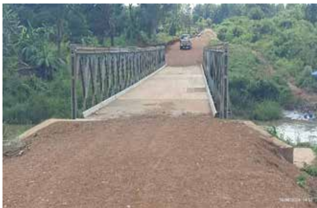
Completed installation of Agwa Bailey Bridge decking in Lira District
