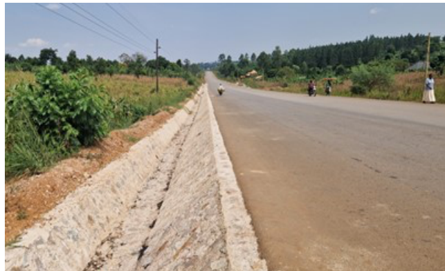
Reconstructed section of Mityana – Mubende road with asphalt and stone-pitched side drains
