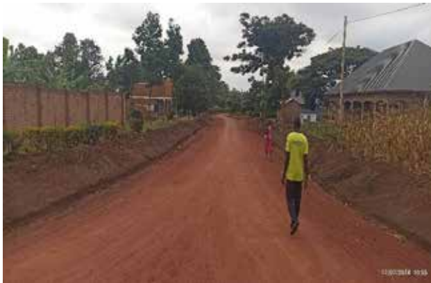
Lira City: A well graded, shaped and graveled section of Temogo road
