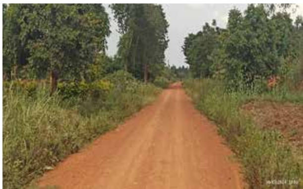
Kwania District: A well-graded and shaped section of Akot-Abwong road at Km 7+400 with overgrown grass on the roadside
