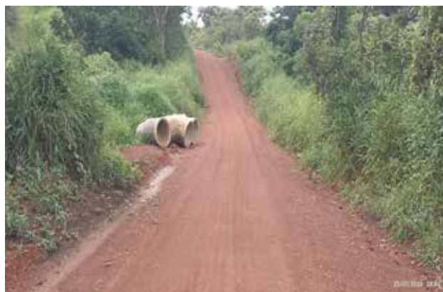
DRRU-North A section along the rehabilitated Tegot Atoo P/S road in Gulu District at Km 1+800 with culverts yet to be installed
