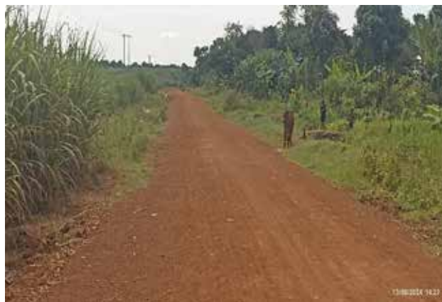
DRRU-Jinja: A well graded, shaped and graveled section at Km 1+300 along the fully rehabilitated Ndalike-Ngandho (2.5km) road in Kamuli District
