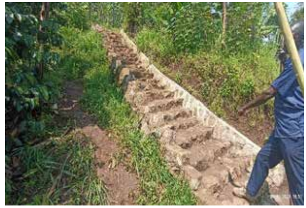
Constructed stone masonry steps that will lead to the metallic ladder in an inaccessible hilly rural area in Namagwi in Bulambuli District
