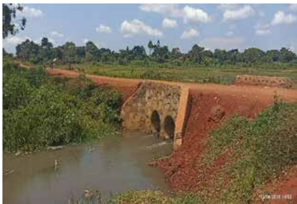
DRRU-Jinja: Installed Armco culverts with end structures in a swamp raised section at Km 4+100 along the fully rehabilitated Ndalike-Namwendwa (6.9km) road in Kamuli District
