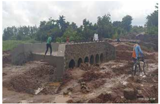
Lira City: Ongoing works of drainage structure with six 600mm diameter culverts at a bottle neck section along the Kulu Owelo (Ongica) road
