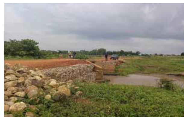
Mbale UNRA Station: Gabion emergency construction works on Kadoto-Butebo road at Km 36+700
