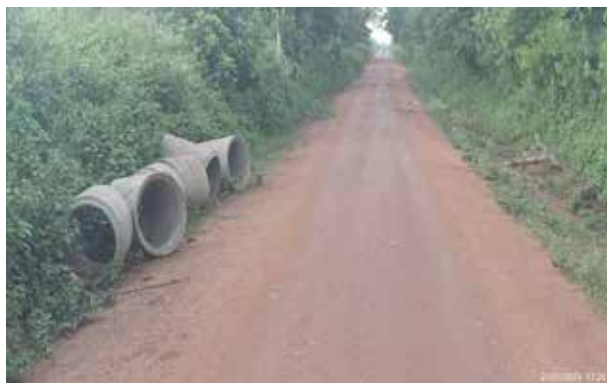
Yumbe district: A well-graded and shaped section of Odravu SS – Yumbe Boma Ground road at Km 12+700 with culverts pending installation
