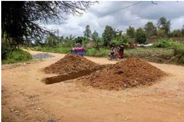
Arua City: Excavation for installation of a culvert along Mvara-Ochiba-Dadamu-Ombachi road at km 3+000
