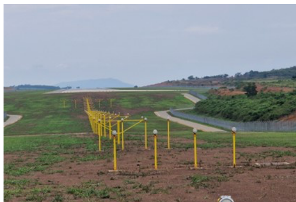
Kabaale International Airport: Airfield Ground Lighting system installed
