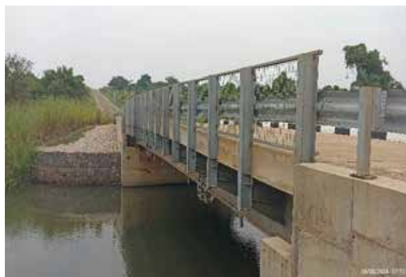
Completed Gazi Bridge along the Inde-Rhino Camp road in Madi Okollo district. Left: The paved approach road works; Right: The bridge structure with the stone pitching and gabion protection works
