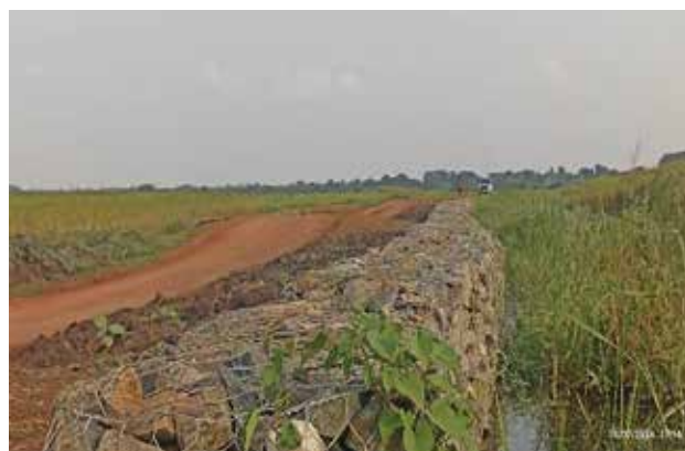
Lira UNRA Station: A section with gabion protection works along Kadilani-Atura-Atapara (23.1km) at Km 2+000
