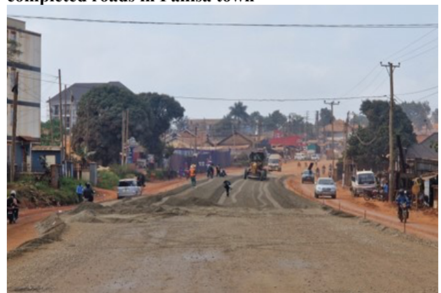
Kira-Matugga Road: construction of base layer along Kira -Kasangati section
