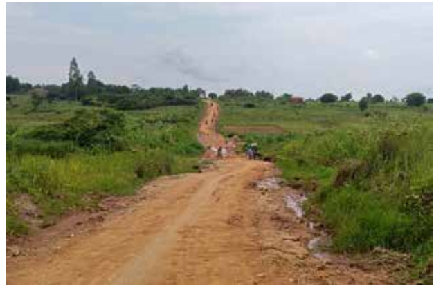
Arua City: A section of Mvara-Oduluba Budrabe road at km 4+900 that was damaged by rain
