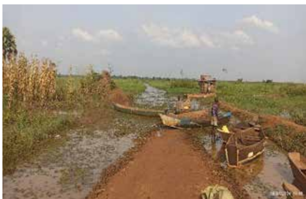
Lira UNRA Station: A flooded section of about 1.8km along the Amii-Kidilani (16km) road at Km 9+000
