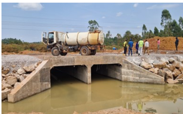
Mityana – Mubende road: Box culvert constructed at km 25 +250
