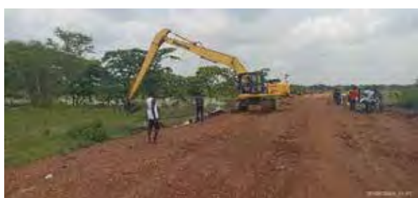
Abarila Swamp crossing on the border of Katakwi and Amuria Districts – ongoing river training
