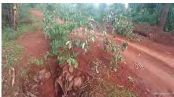
Kapchorwa Municipality: An installed 900 mm diameter culvert line at km 1+000 without end structures on Kapteret–Kaptul–Kabat (4.3 km) under the Road Maintenance Grant
