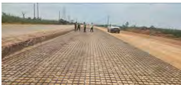
Installation of geotextile material within Lwela Swamp crossing along Kampala–Masaka Road
