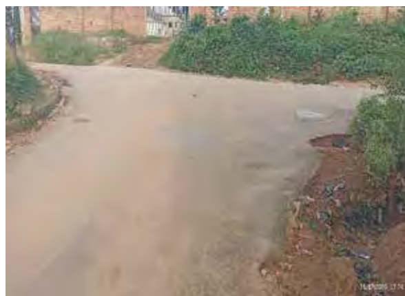
Mbale City: Patch works on Nkokonjeru Court Road (0.2 km) in Namanyoni Ward under URF
