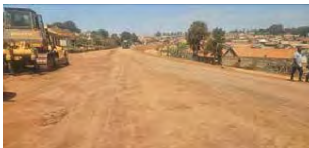
Top of subgrade layer for Masaka–Kyotera Road
