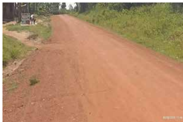
Gulu City: A well graded and gravelled section at km 1+100 along Brother Elio Road (2.5 km) in Bardege Division under the Road Maintenance Grant
