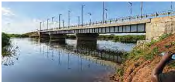
Aleles Bridge in Pallisa District: The bridge structure
