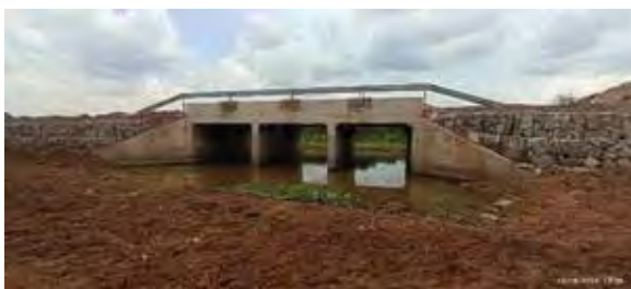
Funguwe-Muwafu Swamp crossing in Tororo District: Left – Three-cell box culvert with gabion protection works
