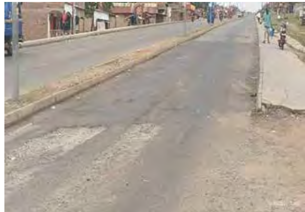
Tororo MoWT Station: Patch works along the Busumbu–Lwakhaka Road at the Lwakhaha border in Namisindwa District done using force account mechanism
