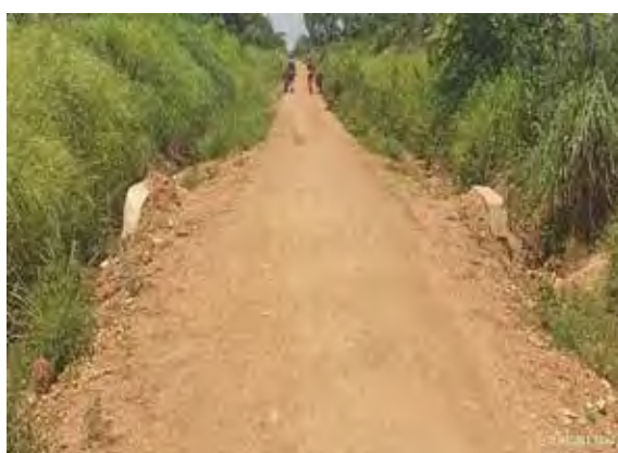
Lamwo District: A well-graded and shaped section with overgrown road grass at km 9+300 along Kitikiti-Paracelle Road (16.1 km) using the Road Maintenance Grant
