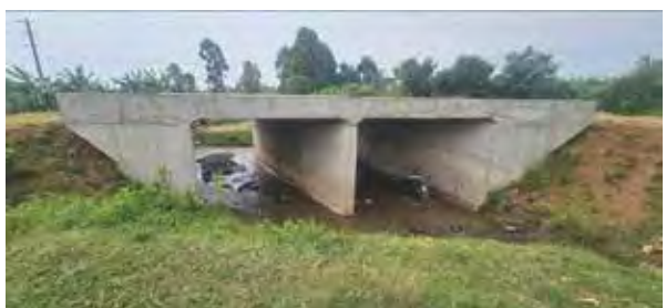
Completed bridge at Mpanga along Ruboni-Bukuku Road with approaches yet to be worked on
