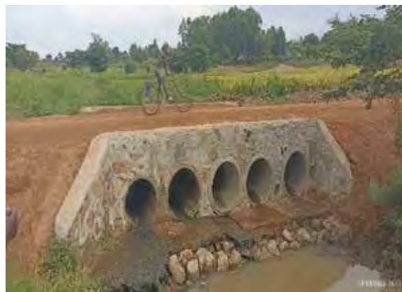
Tororo District: A raised section in the swamp along the Morikiswa–Peipei Road (5.3km) at km 0+800 using the Road Fund Grant
