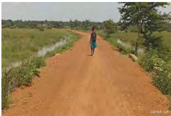
DRRU-East: A section through Akare Swamp at km 2+700 along the Oimai–Arute Road (9 km) in Amuria District
