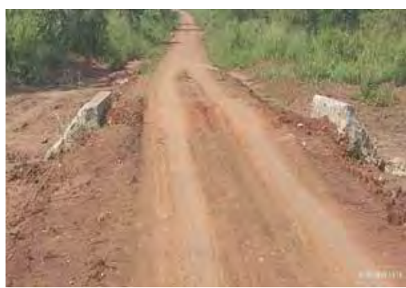
Lamwo District: A well-graded and shaped section with an installed culvert line at km 13+000 along Kamama Central-Apyeta South Road (29.3 km) using the Road Maintenance Grant
