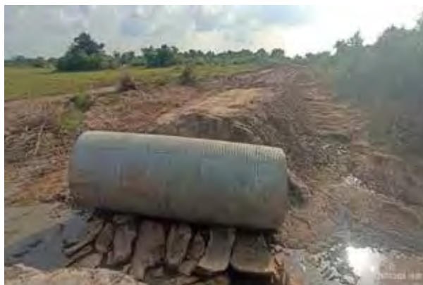
DRRU-East: Ongoing swamp raising and Armco culvert installation works at km 9+000 along the Kapelebyong–Okungur Road (13.4 km) in Kapelebyong District
