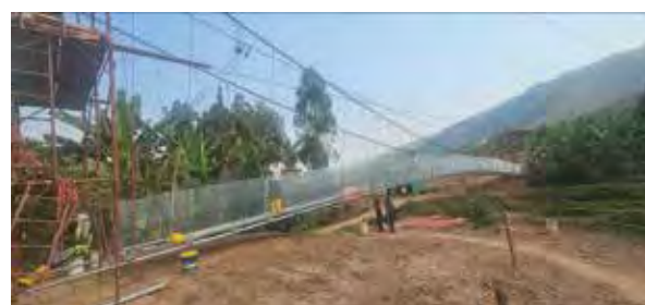
Ongoing construction works at the Nyakeina–Kabira Cable Bridge in Rukiga District
