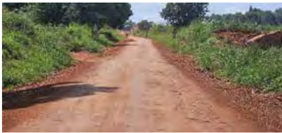
DRRU-West: Left – A completed section of Kyarukoka–Rugoiga–Kihaguzi–Binyinya–Kisaigi road in Kakumiro District
