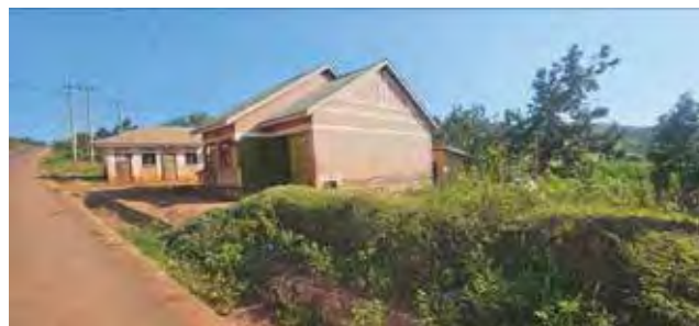
Compensated structures yet to relocate along Kafunta–Buwampa Road in Njeru
