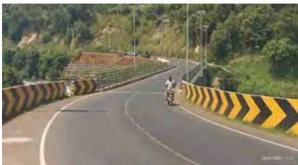
Karuma Bridge along Gulu-Kampala Road: Left – Completed bridge deck with the expansion joints and solar street lights installed; Right – Gabion protection works and preparation for grassing of the embankment
