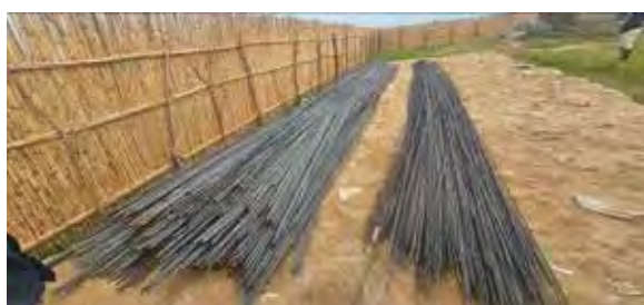
Mobilised materials in preparation for the construction of bridge works at Kiyanja Swamp crossing in Ntoroko District
