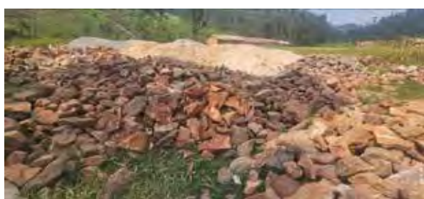
Mobilised hardcore, sand aggregate for the construction of Bikongozo box culvert in Rukungiri District
