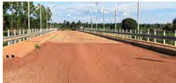
Aleles Bridge in Pallisa District: The deck of the bridge
