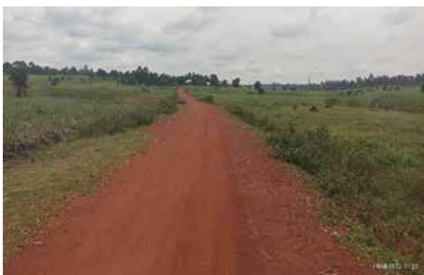
DRRU-Jinja: Left – A well-graded, shaped and gravelled raised section in a swamp at km 3+500 along the Igeyero–Namatolo–Bukapala Road (4.4km) in Jinja District
