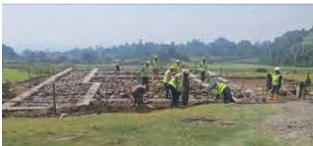
Erection of the site camp for the Kisoro-Mgahinga road link
