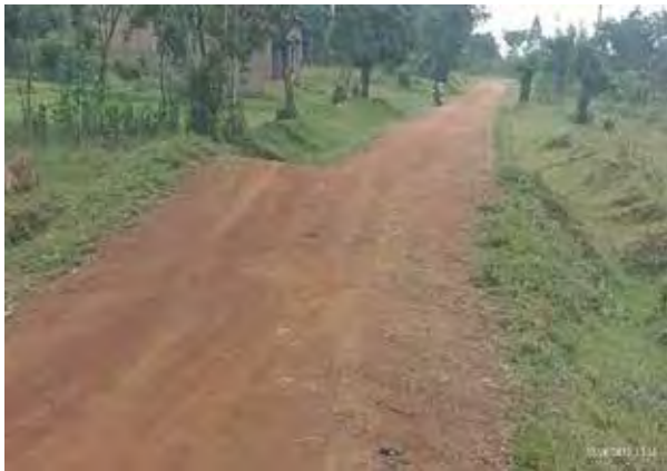
Tororo MoWT Station: A section along the Malaba–Mella–Tuba (26 km) Road with a culvert crossing but no end structures at km 10+500 in Tororo District, done using a framework contract
