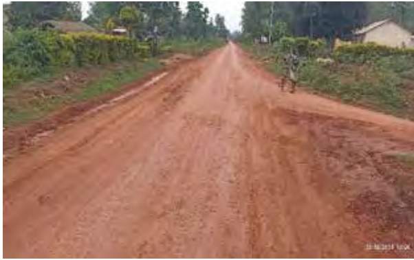
DRRU-North: Left – A well-graded, gravelled and compacted section at km 1+900 along the Teboke–Aboke–Alito–Ogur Road in Kole District
