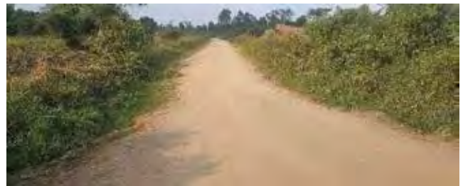
DRRU-West: A completed section along the Kabogore–Ijwara Road in Kazo District
