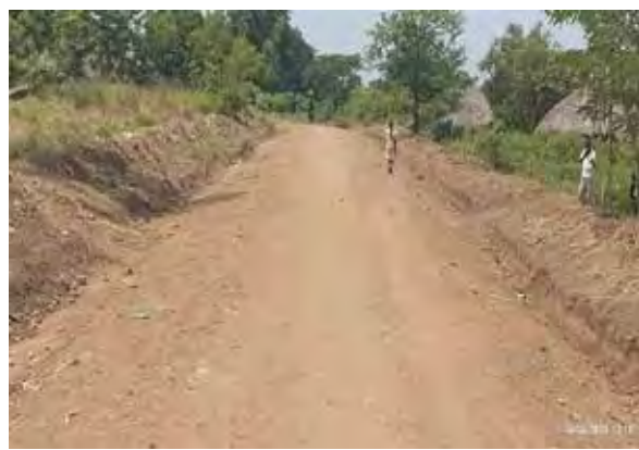
Nebbi District: A graded section at km 3+900 along Rero-Afoda Road (6.8km) using the Road Maintenance Grant
