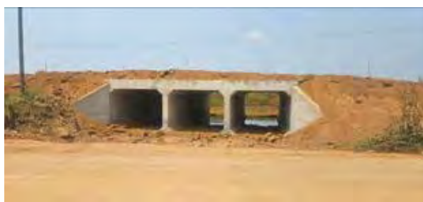
Completed box culvert within Lwela Swamp crossing along Kampala-Masaka Road
