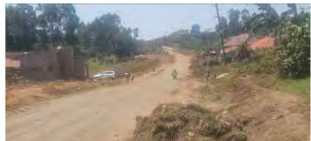
Bush cleared section along the Kabale-Lake Bunyonyi road link
