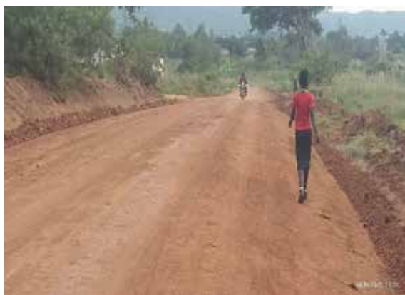
Nebbi District: A well-graded section at km 8+000 along the Nyaravur-Parombo Road (16.2 km) using the Road Maintenance Grant
