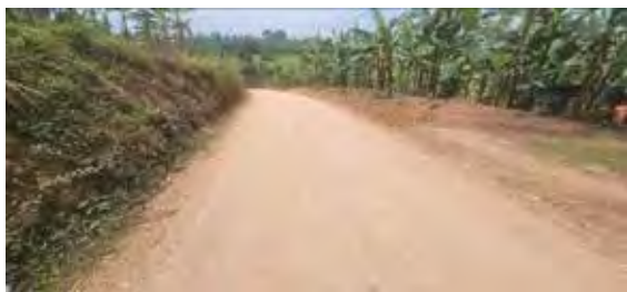
Bushenyi District: Bishop Ogezi Road graded and spot gravelled using the Road Maintenance Grant
