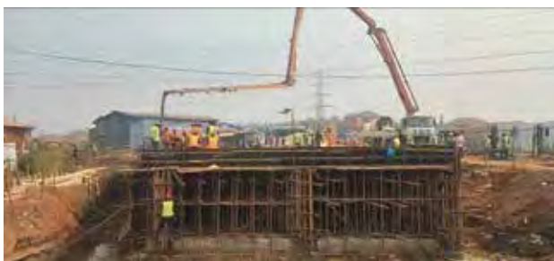
Construction of bridge at Natete along the Natete – Nakawuka Link Road
