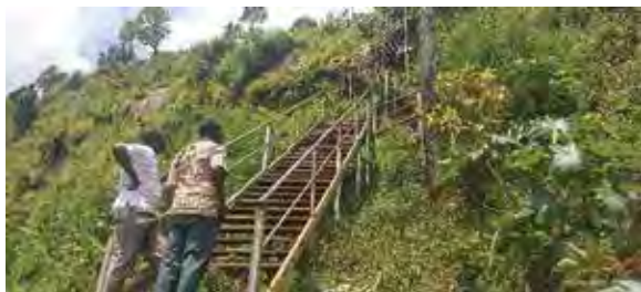
Metallic ladder in Mt Elgon (Namgwi) in Bulambuli District: The steel metallic ladder
