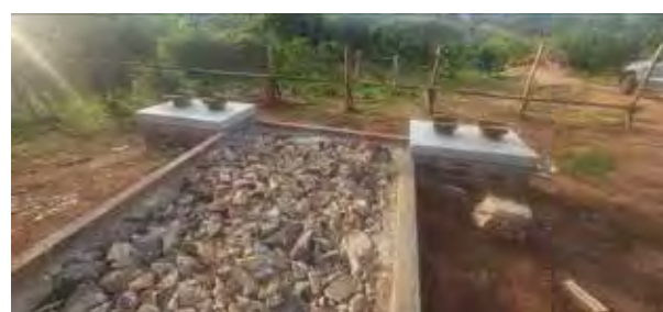
Foundation works for the construction of Haibaale Swamp crossing, Kakumiro District
