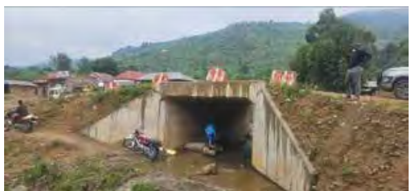
Completed one-cell box culvert at Nyabuswa along the Bukuku-Ruboni Road
