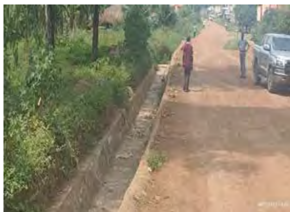
Nebbi Municipality: Drainage improvement works of stone pitching along Pithua Road (1.4km) in Tahata Division under the Road Maintenance Grant
