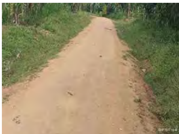
Mbale City: A well-graded and shaped section at km 1+800 along Namanyonyi–Makudyi Road (3 km) under the Road Maintenance Grant
