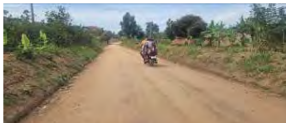
Mubende District: Kasolo–Mugungulu–Nabikakala Road graded section implemented using the Road Fund
