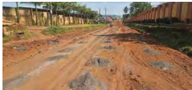
Stabilisation with lime for the base along Mother Kevin and Nsuube Road in Nkonkonjeru
