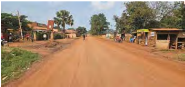
Masindi Station: Gravelled section using force account along the Ihungu–Bulyamusenyu Road
