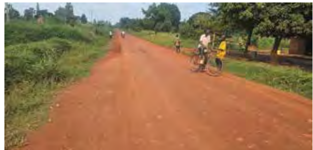
Masindi Station: Gravelled section of the Masindi–Rwenkunya using framework contract
