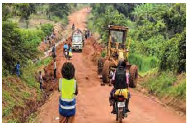
Lira MoWT Station: Spreading of dumped gravel at km 3+700 along Lira–Boroboro–Aboke (41 km) under framework contract
