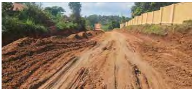
Partially spread gravel for the base works along Mother Kevin and Nsuube Road in Nkonkonjeru
