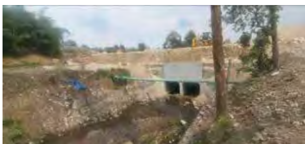
Completed box culvert at the Bwera Bridge
