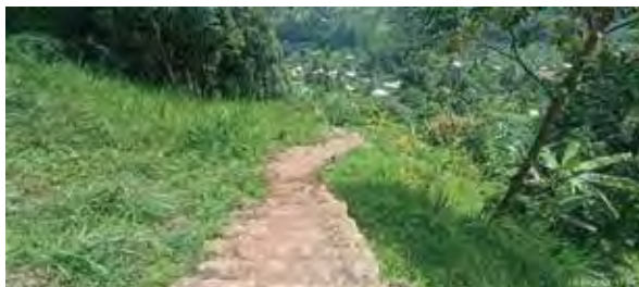
Metallic ladder in Mt Elgon (Namgwi) in Bulambuli District: The stone masonry steps leading to the metallic ladder
