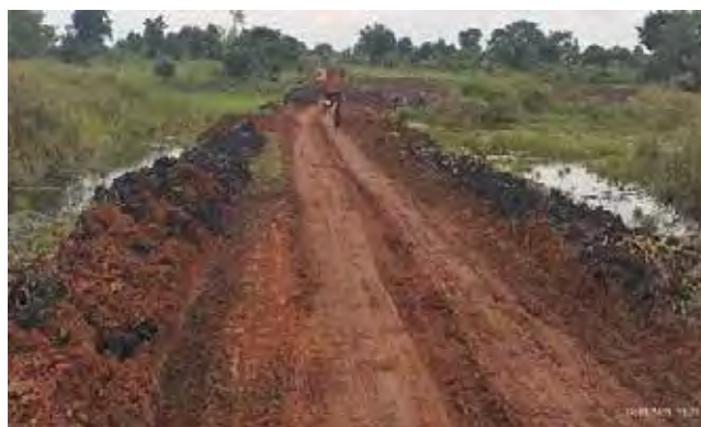
DRRU-Jinja: Ongoing swamp raising works in Naigombwa Swamp (2 km) at the border of Kaliro and Namutumba Districts
