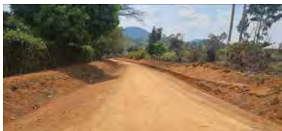
Mubende District: A graded Butawata–Katambogo Road implemented using force account
