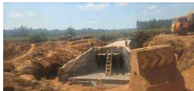
A completed culvert along Masaka–Kyotera Road
