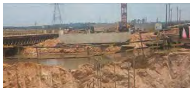
Completed abutment at the Katonga Bridge along Kampala–Masaka Road
