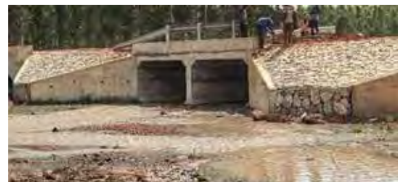
Kadokoleni Swamp crossing in Budaka district: Left – The approach road work; Right– Ongoing works of fixing a guard rail along a two-cell box culvert
