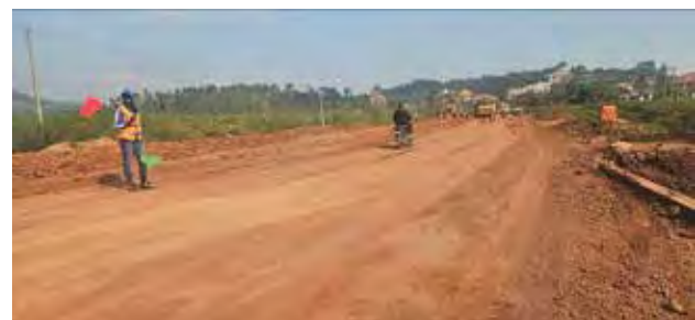
Fill layer up to the top of the sub-grade along the Kisubi – Nakawuka Road
