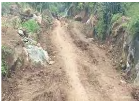
Kween District: An opened and widened section with rock outcrops at km 3+200 on Kapteror-Kapnarkut Road (4.5 km) using the Road Maintenance Grant
