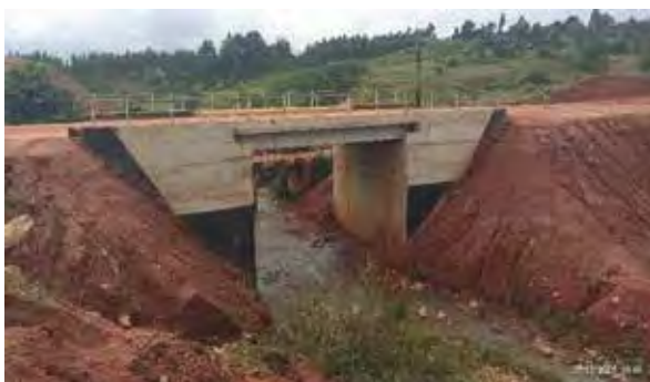
Completed Odrua Bridge structure along Arua-Vurra-Custom-Paidha-Goli Road on the border of Arua and Zombo District
