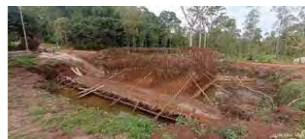
Reinforcement works for the box culvert of Kwapa Bridge project in Tororo District
