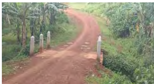
Kapchorwa Municipality: A completed Kaptul Bridge decking at km 4+200 on Kapteret–Kaptul–Kabat Road (4.3 km) under the Road Maintenance Grant
