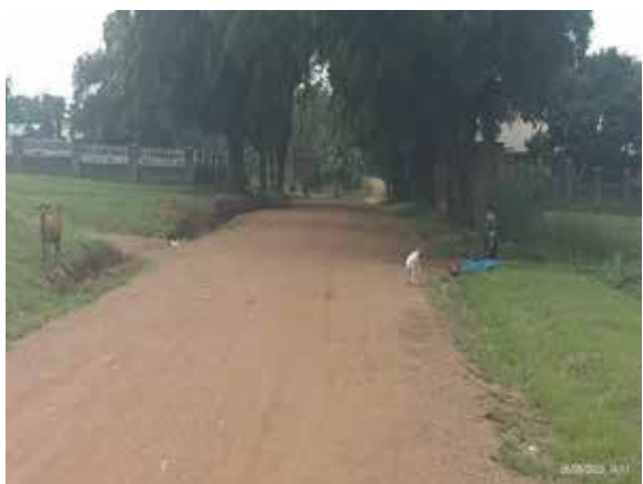
Nebbi Municipality: A well-graded section of Mission Road (0.2 km) in Central Division under URF
