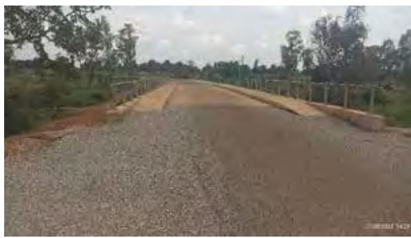
Completed Kochi Bridge structure and the paved approach roads on Keri-Midigo-Kerwa Road in Yumbe District
