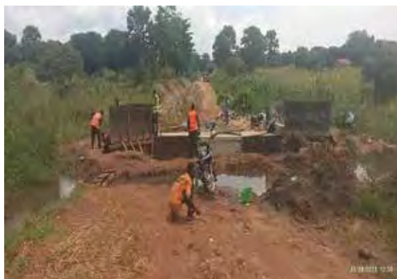
Gulu City: Ongoing drainage construction across Dr. CP Opira Road in Laroo Division under the Road Maintenance Grant
