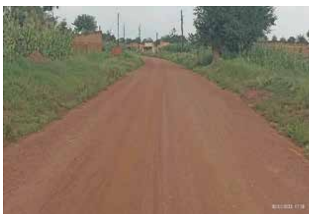
Kitgum MoWT Station: A well-graded and shaped section of Kilak–Adilang Road (65 km) at km 36+300 in Agago District, done using force account
