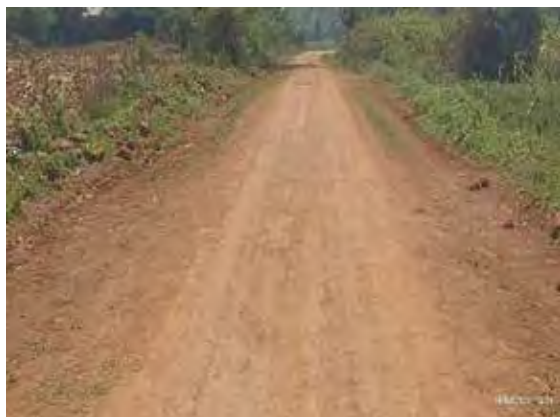
Tororo District: A well-graded and shaped section pending gravelling at km 3 +000 along Iyolwa – Poyem (4.4 km) using the Road Maintenance Grant
