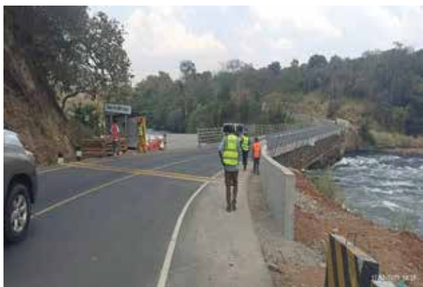
Karuma Bridge along the Gulu–Kampala Road–Olwiyo Road: Left – Newly constructed approach road work to the bridge from Kampala; Right – The newly rehabilitated Karuma Bridge deck with installed guard rails and concrete protection barriers
