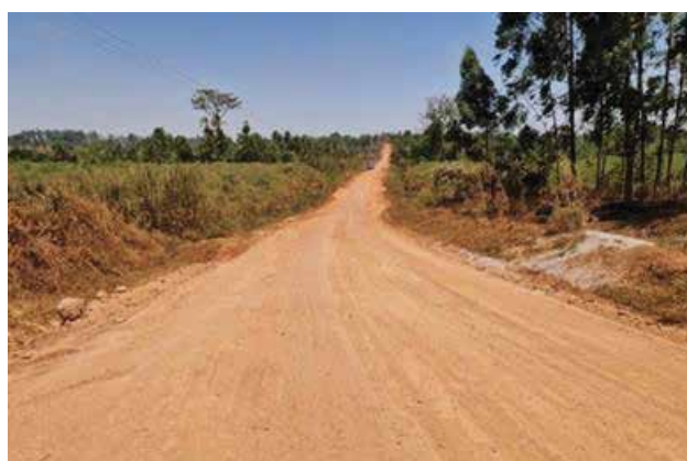
Mubende UNRA station: A section of Nkondo–Malweyo Road (30.1 km) that was gravelled under the framework contract
