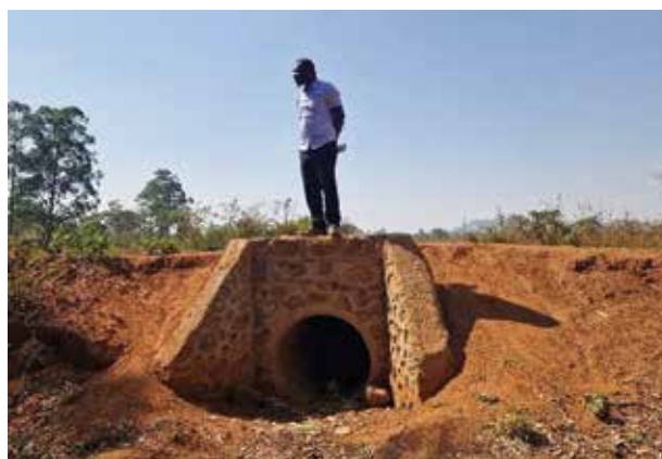
900 mm diameter concrete culvert installed along Bujaja–Kihengamo–Mpasaana Road in Kakumiro District
