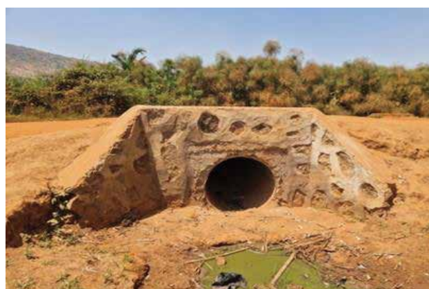
Mubende UNRA station: A 900 mm diameter concrete culvert installed along Nkondo–Malweyo Road
