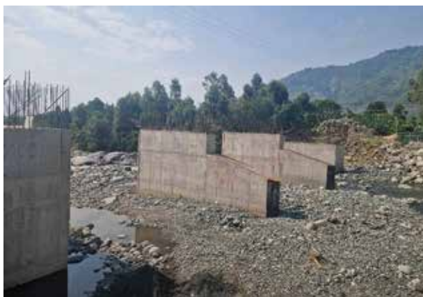
Completed piers and abutments of Kyanya Bridge in Kasese District
