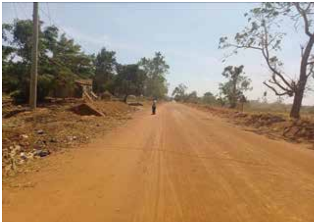
Soroti UNRA station: A well graded, shaped and gravelled section of Soroti–Serere at the start km 16+400
