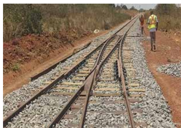
A completed section of the line and a newly constructed turnout at Kumi Station
