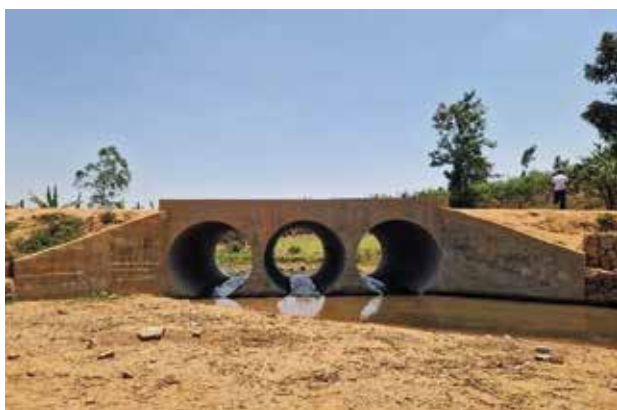
Left–Right: Three lines of 1.2 m diameter Armco culverts were installed along Nyinga–Kalo–Kalungi–Sweswe Road (5.35 km) in Mubende District, gravelled section of the road
