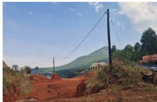
Kabaale International Airport Access Road (3.4 km): Left - Constructed Road Base Layer; Right - Electricity poles in the RoW pending relocation
