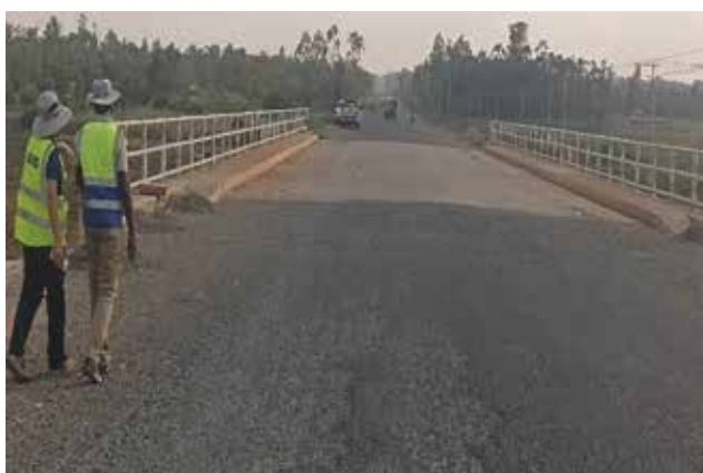
Tororo-Busia Road (26 km): Left – Completed River Malaba bridge with pedestrain walkways and guard rails at km 14+320; Right – Road bed prepatation works towards Busia Town
