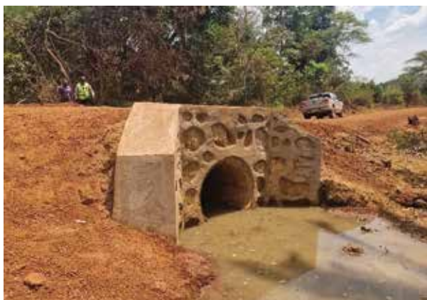
Hoima City: Left–Right: A 900mm diameter concrete culvert installed on Kyentale–Kikwatamigo Road (10.1 km), gravel dumped along the Buswekera–Kaitira–Kihukya–Nyarugabu Road (10.1 km), awaiting spreading and compaction
