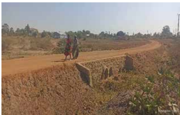
A culvert crossing complete with headwalls at km 0+200 along Oluka Road in Soroti City
