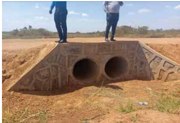
Soroti UNRA station: A double culvert crossing of 900 mm diameter complete with headwalls installed along Soroti-Serere at km 17+400
