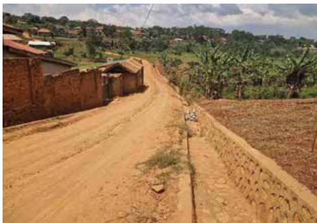
Kawuga–Grammar Road (1.0 km) in Mukono Municipality. The road suffered gravel loss
