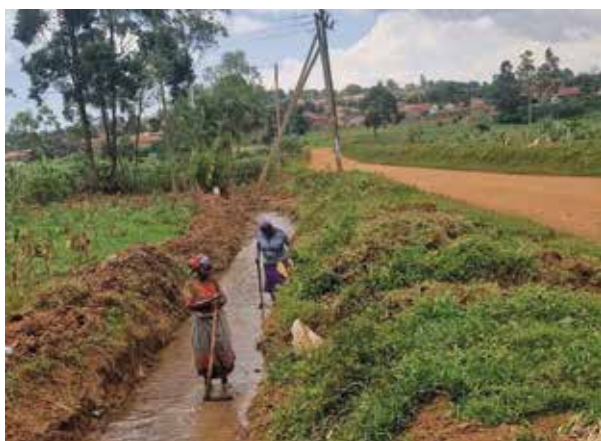
Mukono MC: Road gang undertaking routine manual maintenance with no personal protective equipment (PPE)
