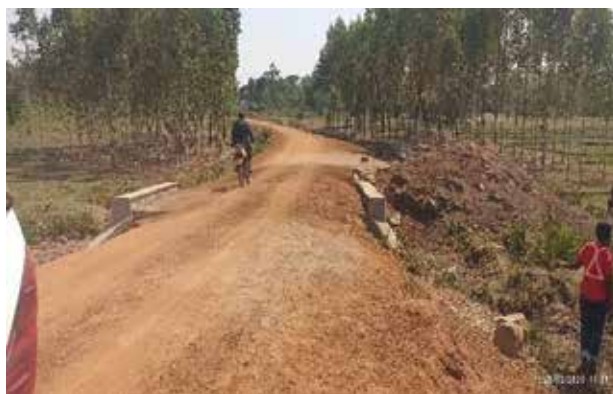
A culvert crossing complete with headwalls at km 2+300 along Senda–Abari–Nagoke Road (9.0 km) in Tororo District
