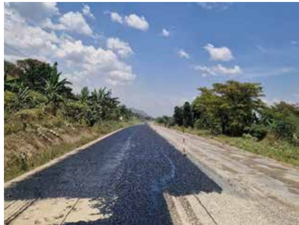
Busunju–Kiboga–Hoima Road: Priming of the base layer in preparation for the asphalt layer
