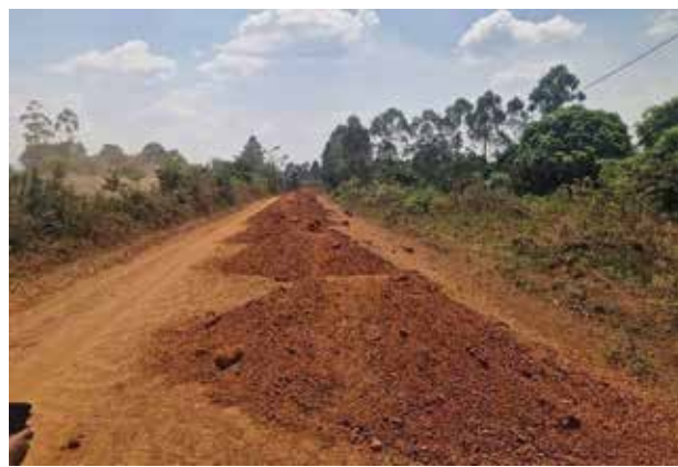
Hoima City: Left–Right: A 900mm diameter concrete culvert installed on Kyentale–Kikwatamigo Road (10.1 km), gravel dumped along the Buswekera–Kaitira–Kihukya–Nyarugabu Road (10.1 km), awaiting spreading and compaction
