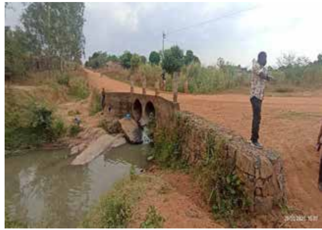
Arua UNRA station: A bridge along the Arua-Muni PTC Road where gabion protection works were done
