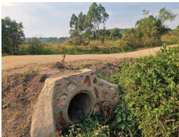
Mubende District: Left-Right: A 600 mm diameter concrete culvert installed on Dyangoma–Bubanda Road as part of the maintenance works in Q2; gravelled section of Dyangoma–Bubanda Road
