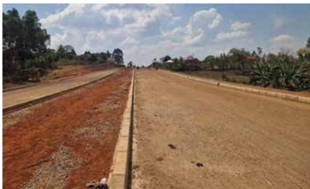
Kabaale International Airport Access Road (3.4 km): Left - Constructed Road Base Layer; Right - Electricity poles in the RoW pending relocation
