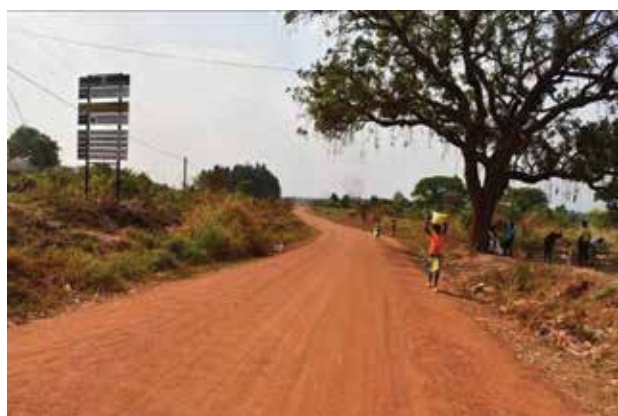
Gulu UNRA station: A well graded and shaped section of Amuru–Omee–Rhino Camp ( 53 km) Road) at km 0+000
