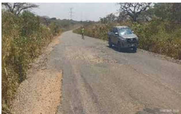
Karuma-Olwiyo Road: A deteriorated section at km 4+900 that had been worked on
