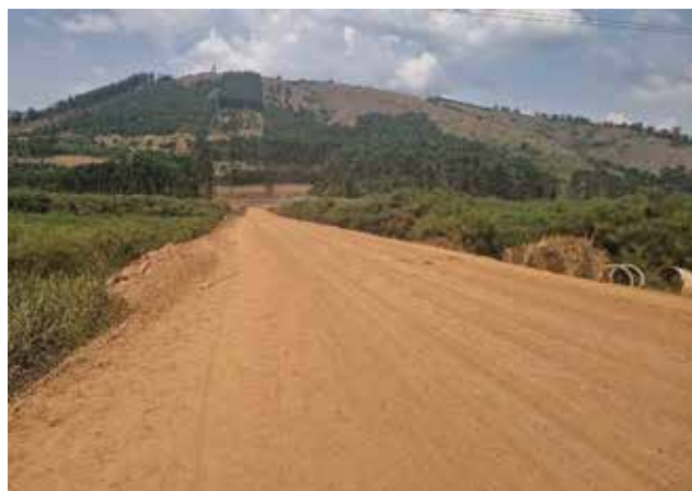
Mbarara UNRA station: Rwoho Swamp was raised as part of the maintenance works under the framework contract
