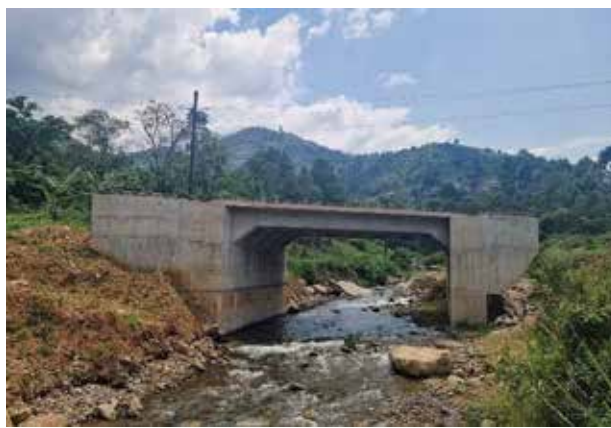
Completed deck of Isango Bridge in Kasese District
