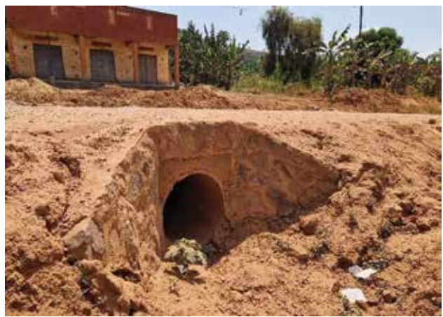
Masaka UNRA station: Left–Right: Graded section of Lumbugu–Lyantonde Road (50 km), 900 mm concrete culvert installed on the road
