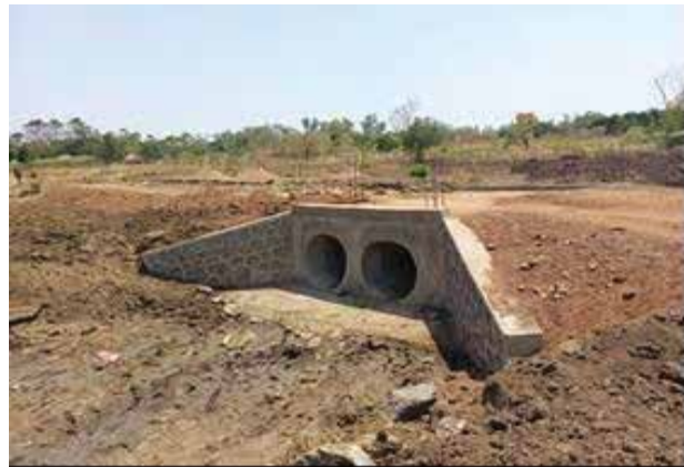
Terego District: A bridge of 1.5 m diameter Twin Armco pipe culverts installed at km 0+300 along Amania–Issa Road
