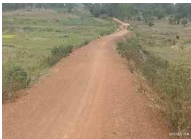
A swamp raised section along Kirerema–Kigalama HC Road (3.7 km) at km 2+600 in Namutumba District
