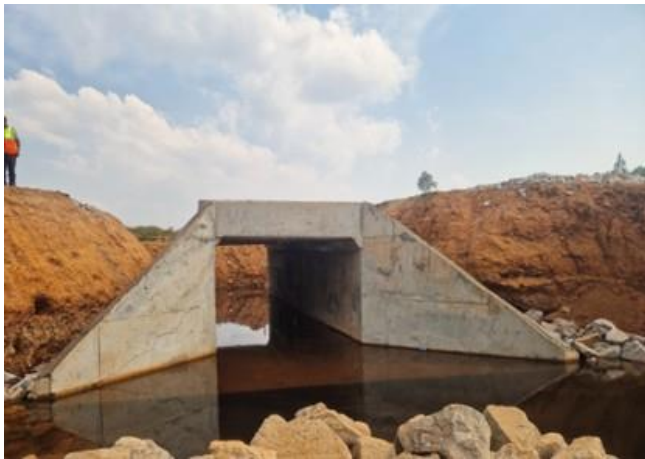
Busunju–Kiboga–Hoima Road: Completed single-cell box culvert
