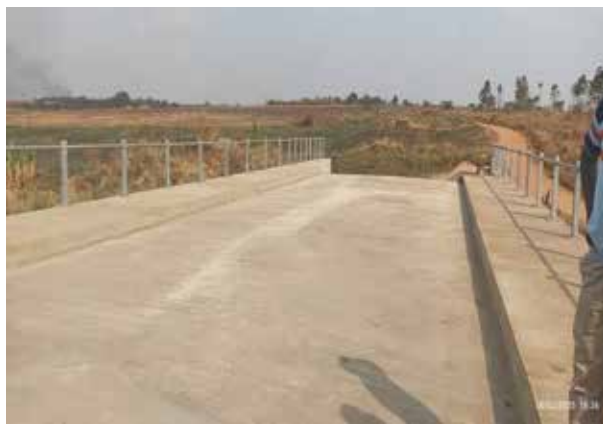
Apaa Bridge on the Amuru–Omee–Rhina Camp Road in Amuru District: Left – Bridge Structure; Right - Top of the bridge deck with pedestrian walkways and railings on both sides
