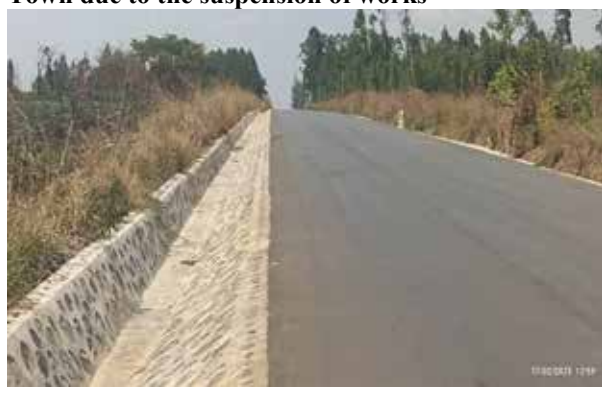
Karuma-Olwiyo Road: A completed section with a stone-pitched side drain at km 42+000
