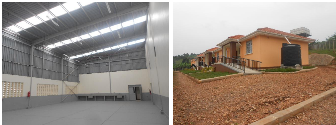
L-R: The completed but not yet fully equipped plant house; and a view of the completed staff quarters at Rwengoma, Ntungamo District
