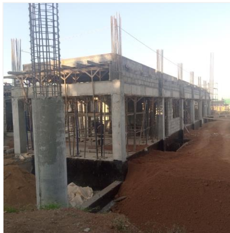
The National Water Quality Laboratory under construction at Entebbe
