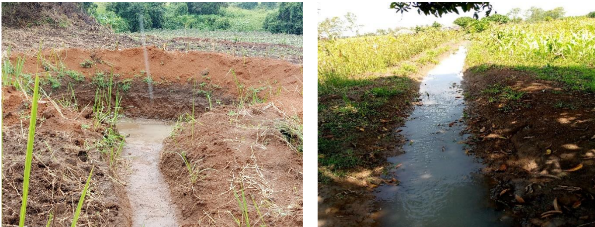
Left: Percolation pit in Koboko district; Right: Flood control trench covering three villages of Ajara, Ogwo and Pece in Patongo town council Agago district
