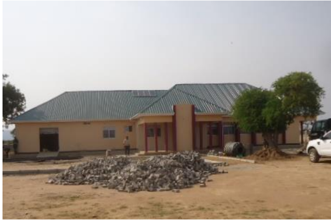
Lakes George and Edward Surveillance Station at Kaiso, Hoima District
