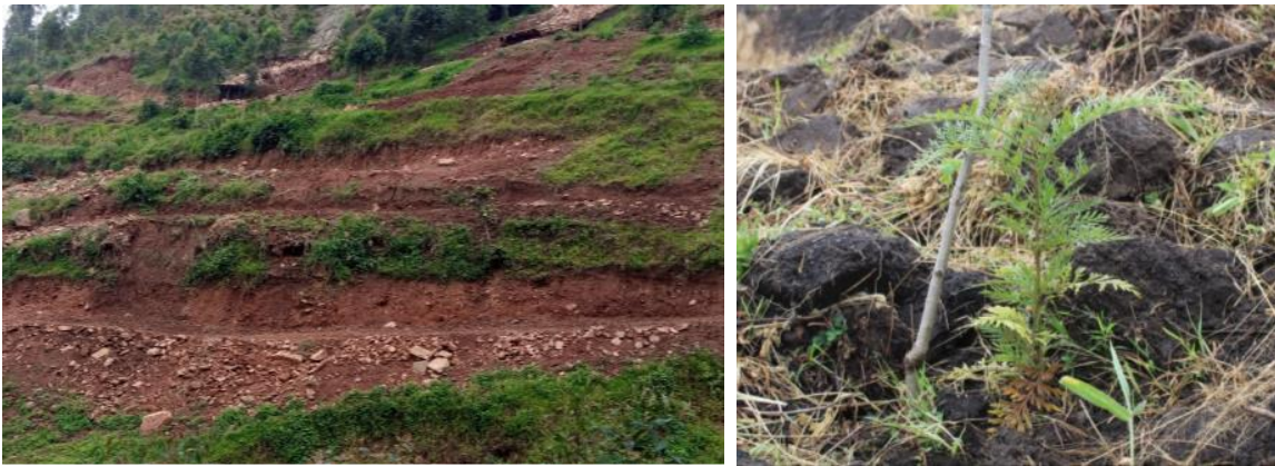
L-R: A bench terrace in Kibuga Parish, Kasese District and gravellier seedling in Nyakitokoli Parish, Kabarole District
