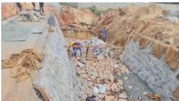
L-R: Stone pitching along a road in the North Estate. A levelled A2 road ready for paving in South A Estate of the Kampala Industrial and Business Park
