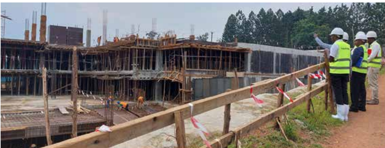
Construction of the National BDS Centre at Butabika-Kampala
