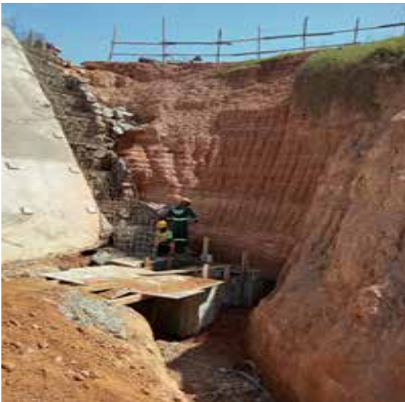
L-R: Completed embankment wall and ongoing works for the cascading storm channel at Entebbe International Airport Free Zone
