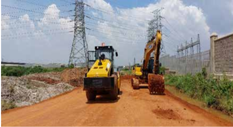
Ongoing road works in South B estate, KIBP-Namanve
