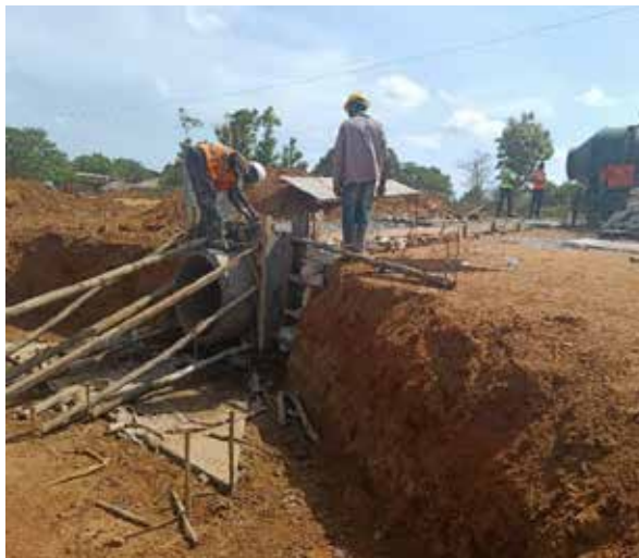
Concrete encasing works on the pipe culvert at km 39+660 along Moyo-Yumbe-Koboko Road
