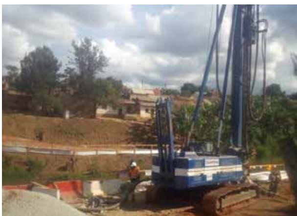
Micropiling works at R. Rwizi Bridge crossing in Mbarara
