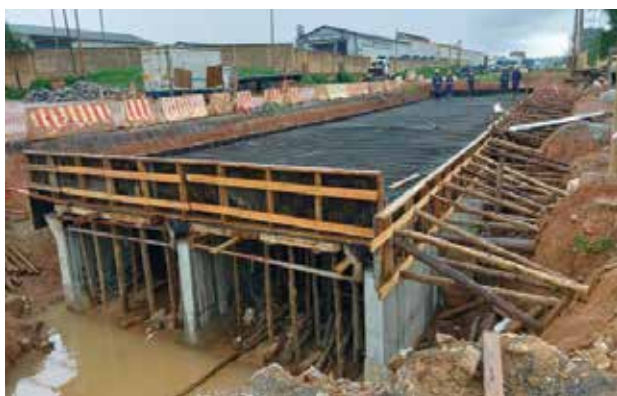
L-R: A box culvert along A3 road in the South A Estate. Drainage works along a road in the North Estate, KIBP, Namanve.
