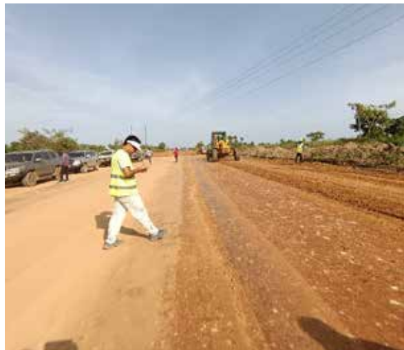
Levelling of the sub-base material at km 14+781 along Moyo-Yumbe-Koboko Road
