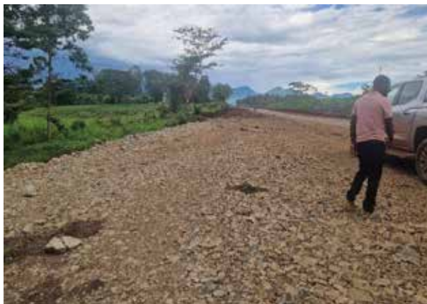
Namagumba–Budadiri–Nalugugu Road, L-R: Rock filling of a swamp section at km 7+475; concrete plant assembled at the contractor's camp in preparation for concrete works
