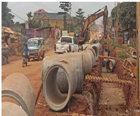
Ongoing 900 mm diameter concrete pipe culvert installation works at km 6+900 along Cyprian Kizito Road in Kira Municipality
