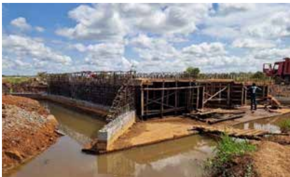
Construction of a 3-cell box culvert across Ibuje Swamp at km 72+100 along Rwenkunya – Apac Road Project
