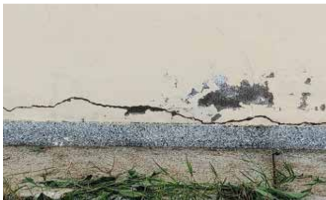
L: A functional PSP for Palabek-Kal WSS in Lamwo District; R: Cracks on the public latrine wall for Lacekocot WSS in Pader District
