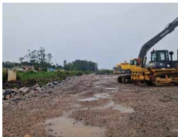
Busega-Mpigi Express Road Project: Left – Construction of abutments at interchange 1 (IC 1); Right – Rock filling of the swamp section along link road 1 at Km 0+940
