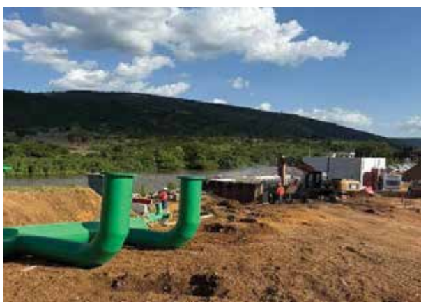
Pipe connection to the raw water pumping station (intake works) at Nzingezi, Kagera
