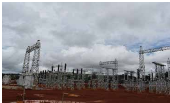
Installed power transformers, erected equipment structures and busbar gantries in the Buloba substation switchyard
