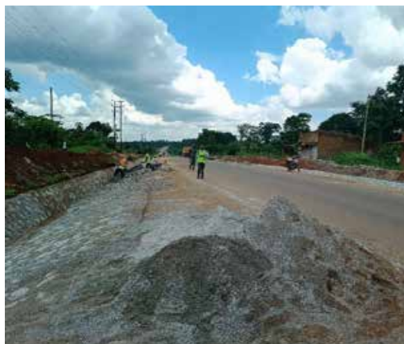
Stone pitching works on a finished pavement section at km 9+170 along the Luweero-Butalangu Road
