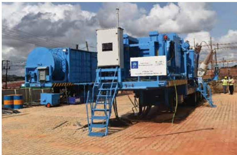
MV trailer and HV trailer for the 132/33 kV mobile Kawaala substation
