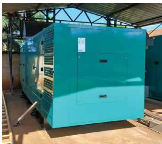
Left: Installed equipment at the MAN Centre in Kampala. Right: A 250kva generator for the Data Centre in Jinja.
