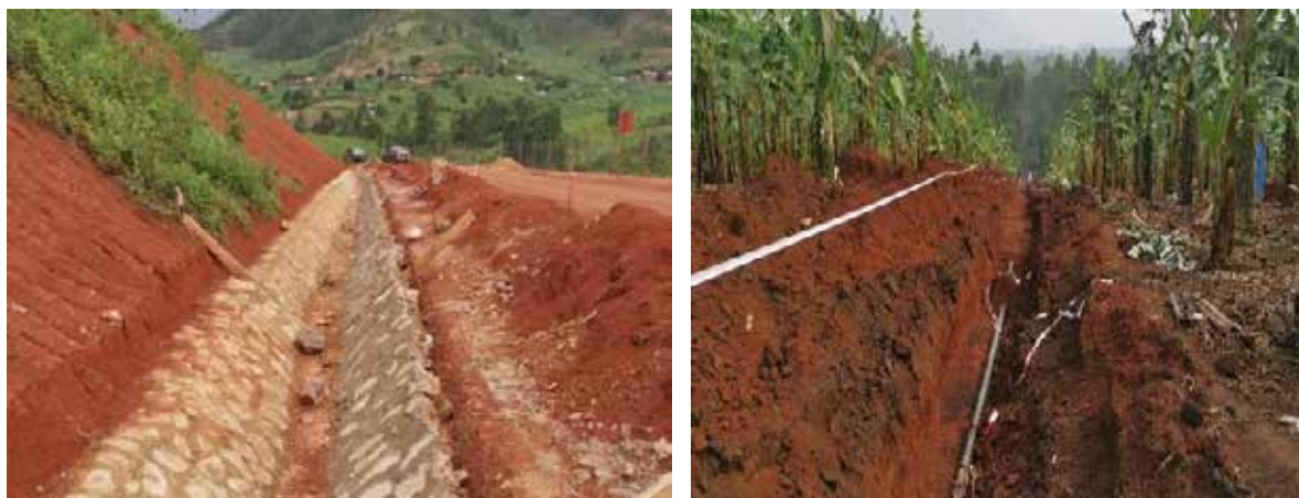
Stone-pitched drainage under construction and pipe laying in Kabuyanda, Isingiro District
