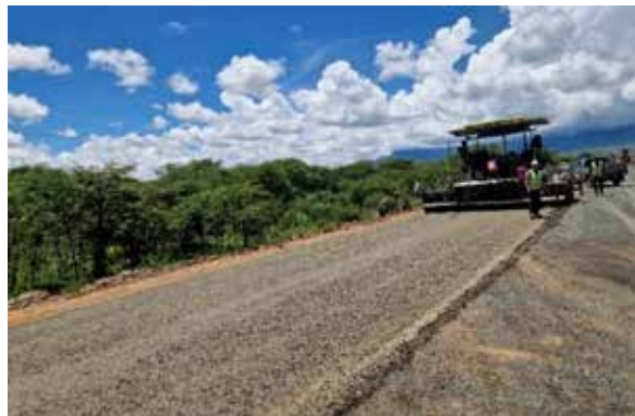
Muyembe–Nakapiripirit Road Project: L – Laying of base layer at km 74+800; R – Completed Chepsikunya Bridge at km 42+170
