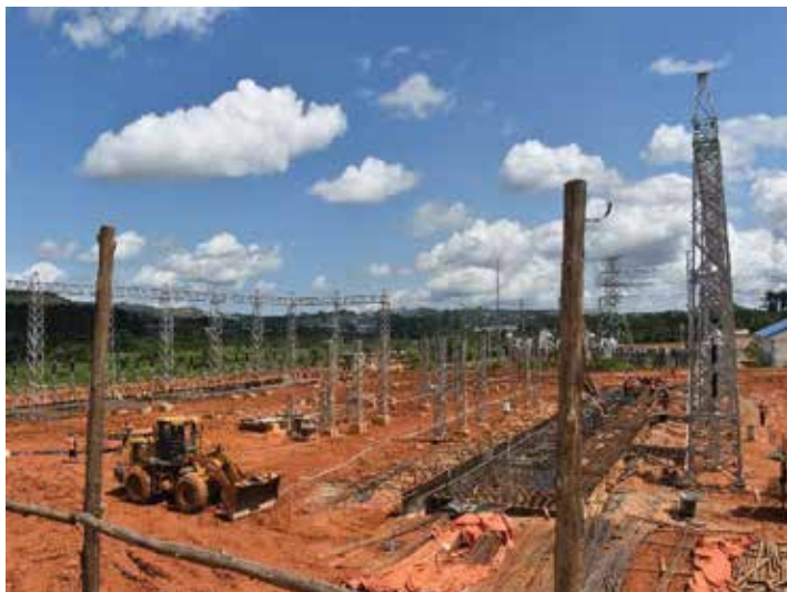
Completed busbar gantries and ongoing foundation works at Mukono substation
