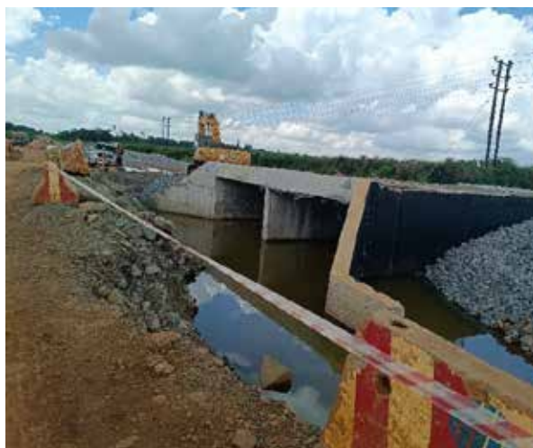
A box culvert at one of the swampy sections along Luweero-Butalangu Road
