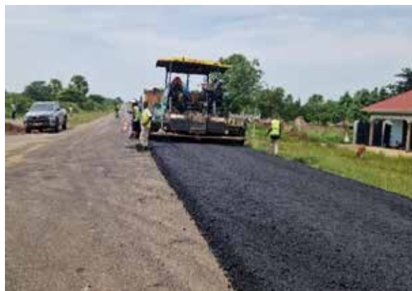
NERMP: Laying of dense bituminous macadam along the Soroti– Lira Section at km 24+400
