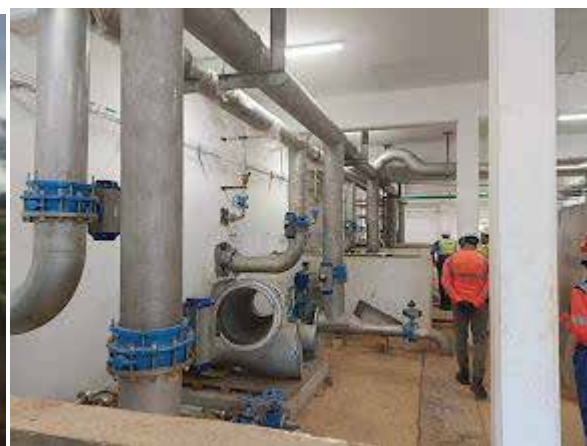
Electrical and mechanical installation at the drinking water pumping station at the Kagera waterworks
