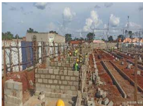
Ongoing works of walling and foundation for the lock-ups and stalls, respectively, at Kigumba Market
