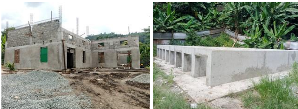
L: The chemical mixing house; R: Stud columns awaiting the reservoir tank at Nyamugasani WSS in Kasese District
