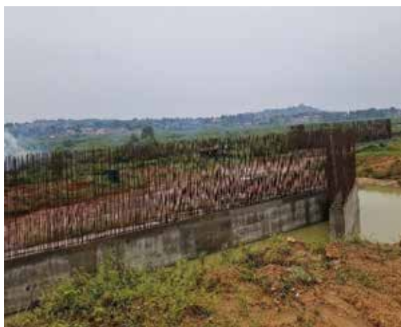
Busega-Mpigi Express Road Project: Left – Construction of abutments at interchange 1 (IC 1); Right – Rock filling of the swamp section along link road 1 at Km 0+940
