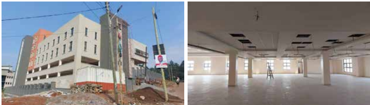
L: A substantially completed Business Development Services (BDS) Centre in Butabika. R: The conference area of the BDS Centre in Butabika, Nakawa Division, Kampala City.
