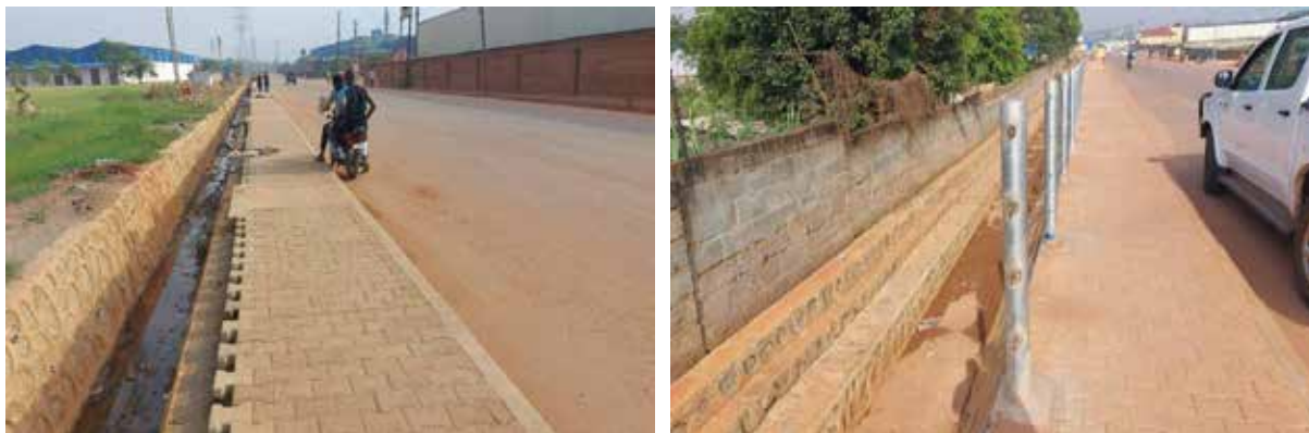
L-R: A nearly completed walkway and drainage channel. Guardrail installation in the North Estate of the Kampala Industrial and Business Park, Namanve, Mukono District.
