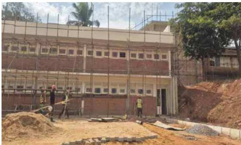
Ongoing renovation works at the Uganda Museum, Kampala City.
