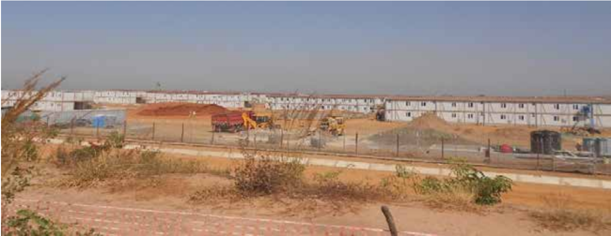
Ongoing construction of workers housing facilities at the Tilenga CPF site
