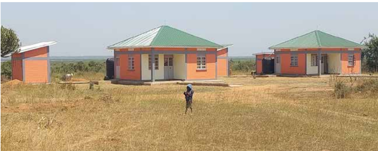
Completed resettlement houses for PAPs displaced by Tilenga flow lines in Kirama village, Buliisa district
