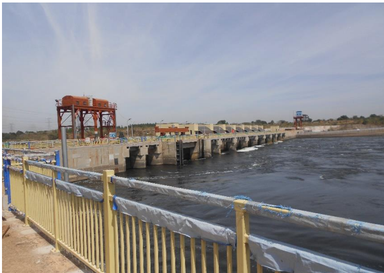
Ongoing works on the safety barriers at Karuma HPP
