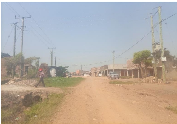
Completed grid extension scheme under UREAP Lot 2 in Lugungudde TC, Wakiso District
