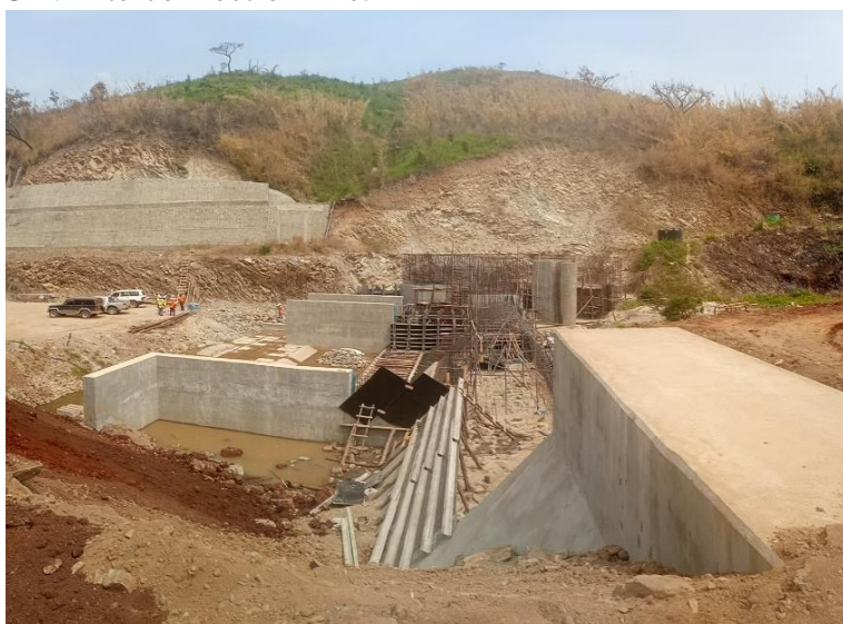
Ongoing civil works at the Nyagak III dam intake
