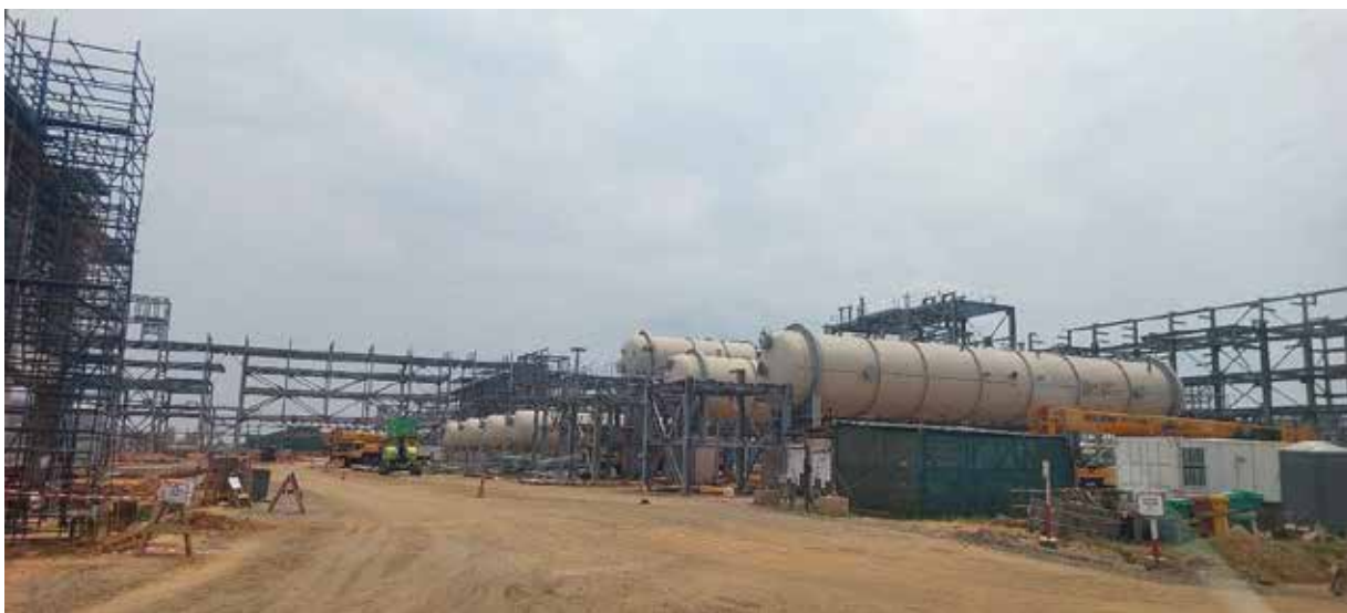
Ongoing civil and electromechanical works at the Tilenga CPF site in Buliisa
