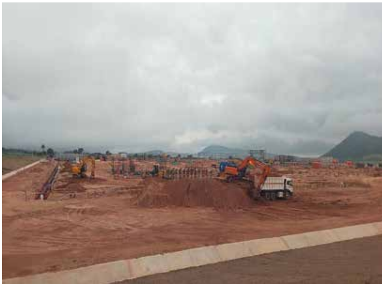
Ongoing civil works at EACOP Pumping Station (PS1) in Kabalega Industrial Park, Hoima District
