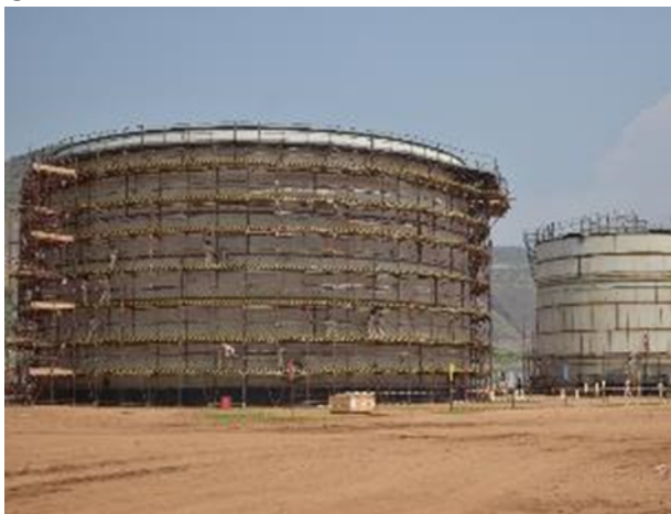
Works at the crude on-spec and off-spec oil storage tanks at the Kingfisher Central Processing Facility
