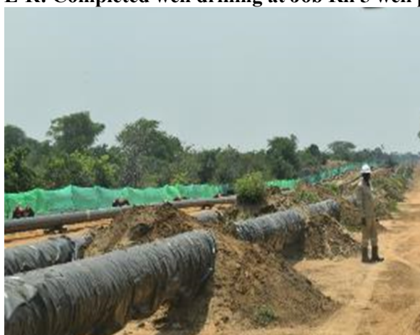
L-R: Flow line pipe laying from Job Rii to the CPF; Early civil works at the cellar pit at Ngiri 5 well pad
