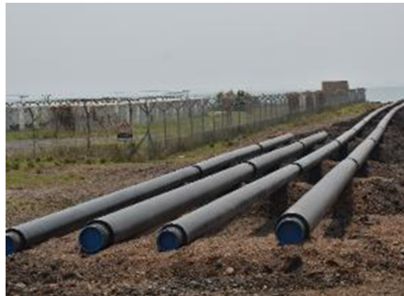
L-R: An operational rig at well pad 1; Flow line pipe laying works from the well pad 2 to the CPF
