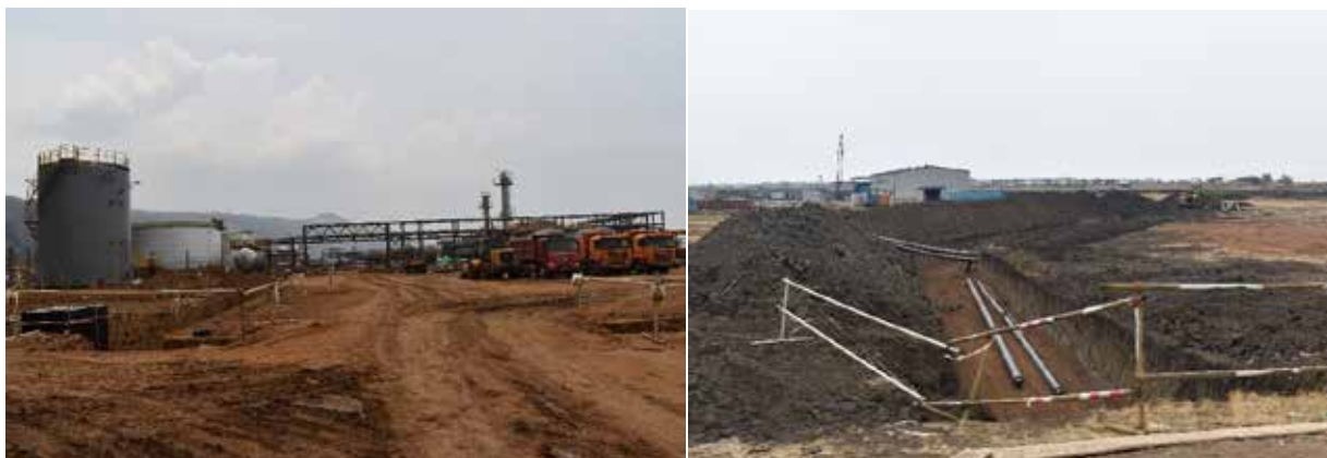
L-R: Ongoing works at the on-spec, off-spec and crude oil pig receivers; Flow line pipe laying works from well pad 2 at Kingfisher, Buhuuka Village.
