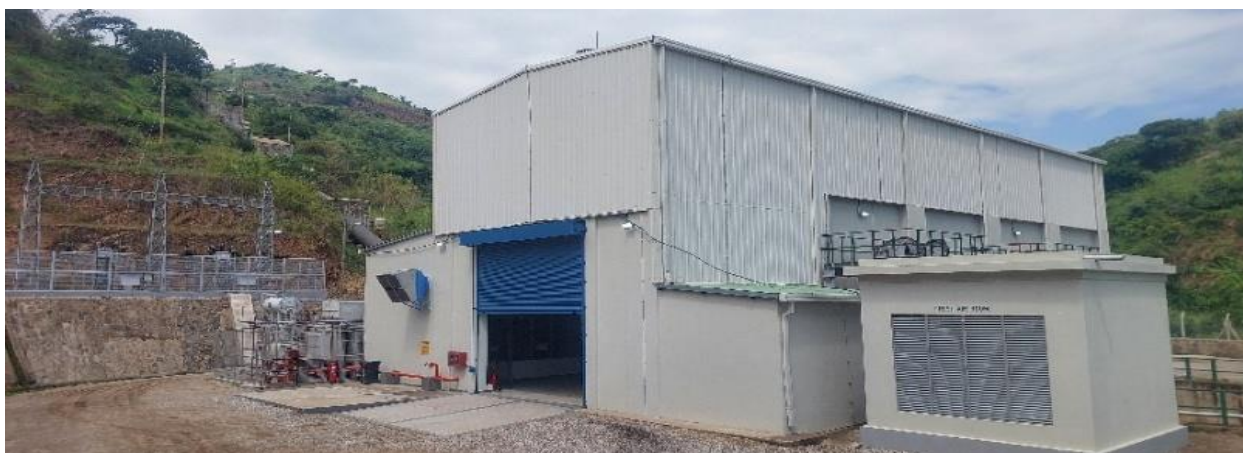
Completed Nyagak III power house building
