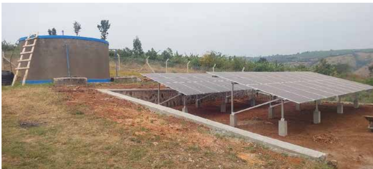
Completed solar water supply scheme at Ntungu, Isingiro District
