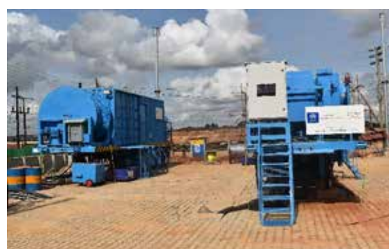
L-R: Ongoing construction works at the 132/33 kV Buloba substation; installed mobile substation at Kawaala
