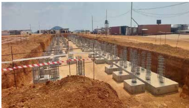
Ongoing foundation works at Kabaale substation in Hoima
