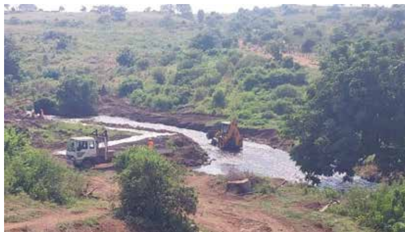
River diversion works at the Hoimo mini-hydro site, Hoima
