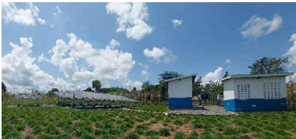
Completed solar water supply scheme at Purongo in Nwoya District
