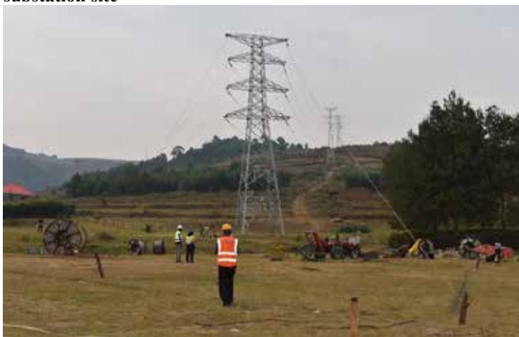
Stringing of the conductors on the Kabale-Mirama Transmission line at Bukinda, Rukiga District.
