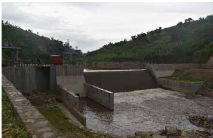
Completed dam and spillway structure at the Nyagak III HPP
