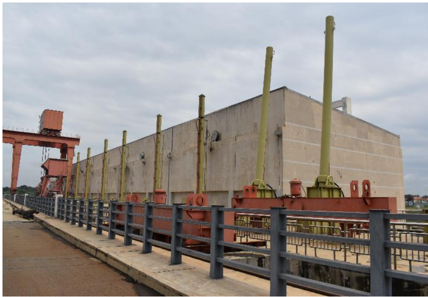
Plant house building and gate lifting hydraulic actuators at the Isimba HPP
