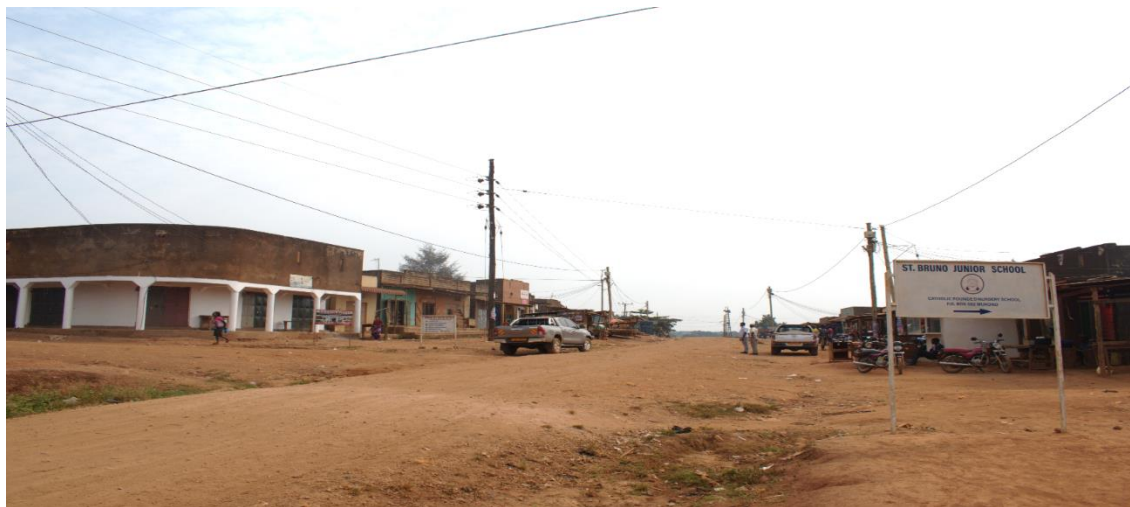
Completed grid extension scheme in Kiwumu TC, Mukono District under ERT III
