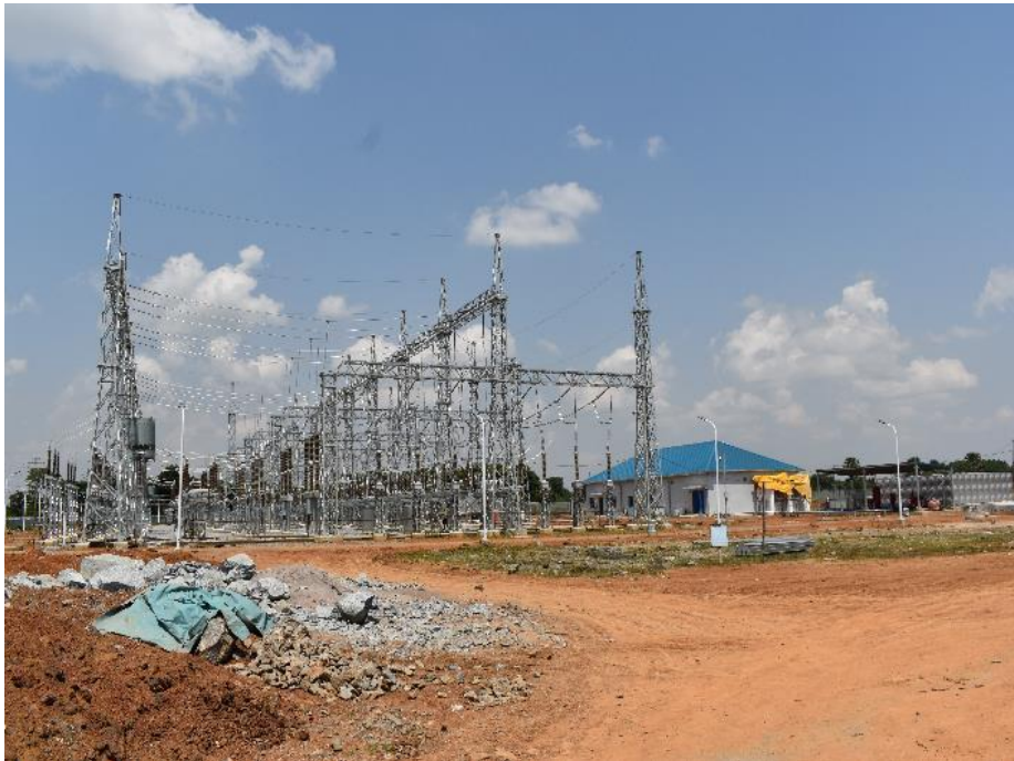
Completed plant house building, equipment structures and busbar gantries in the new 132kV Kole switchyard
