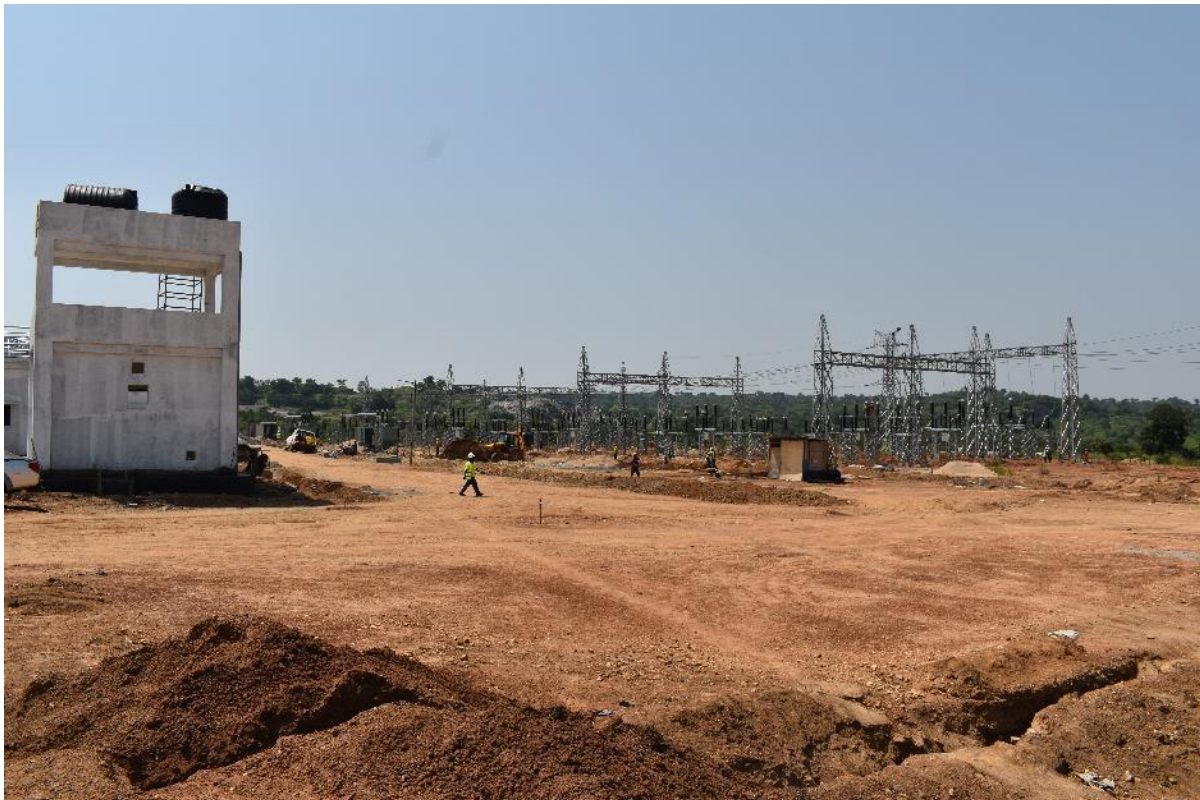
Ongoing works at the 132kV Agago substation
