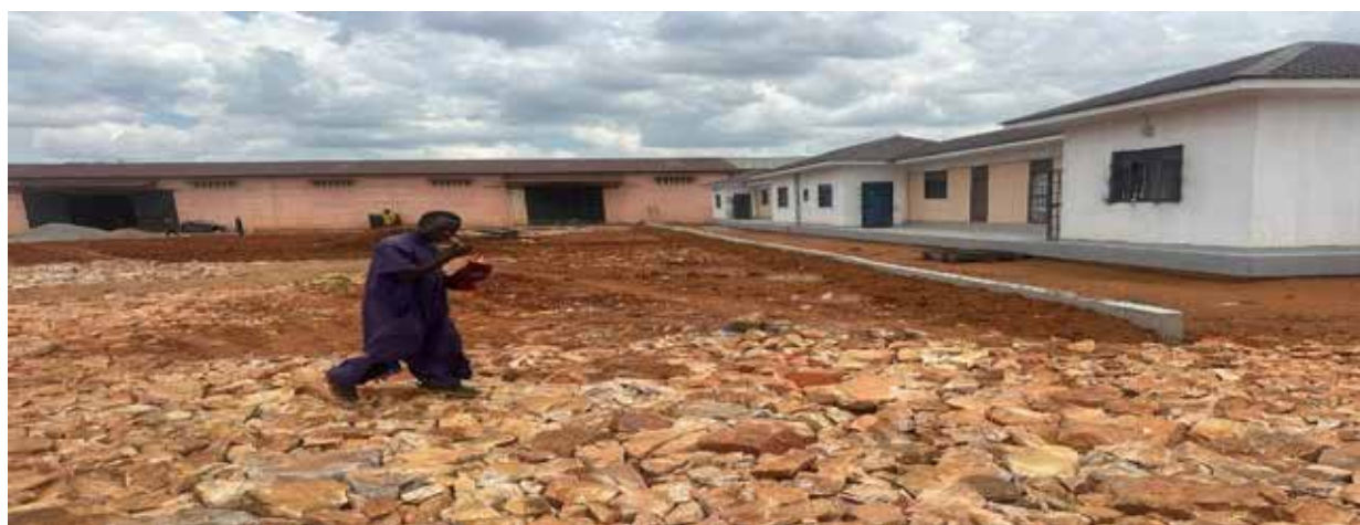
The yard is near completion
