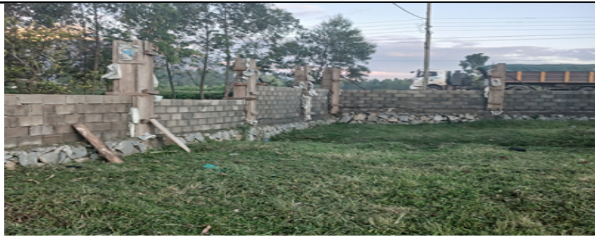
Different views of the perimeter fence that was constructed by the Ministry around the mechanisation centre
