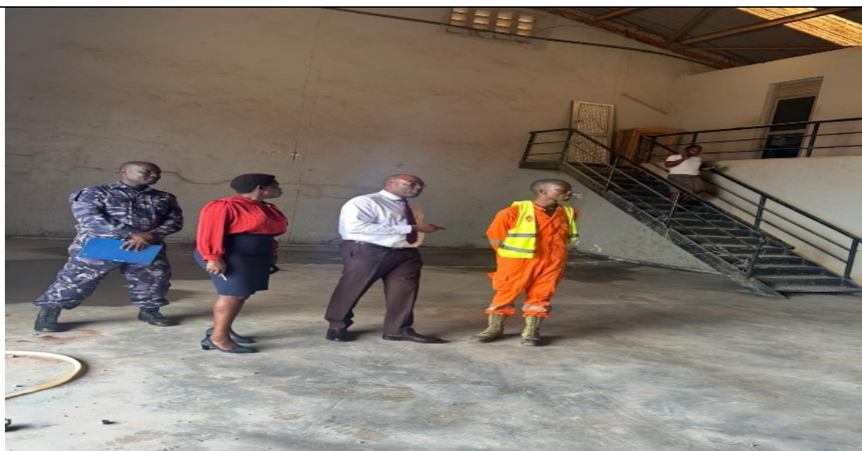
Warehouse: Inspection of the completed works on the floor
