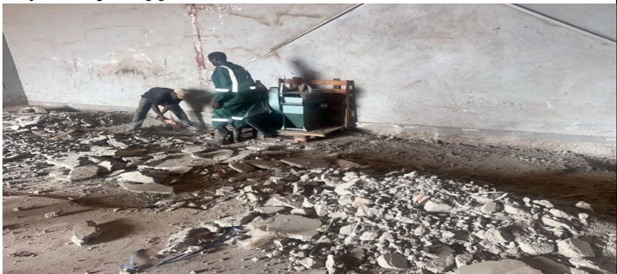
Excavation of the floor in the main store
