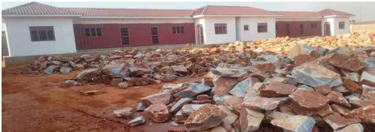
20 40ft Containers fabricated into offices and completed. Hardcore is being placed to reinforce the parking yard
