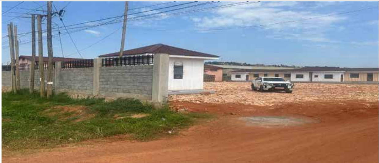
View of premises with perimeter wall completed, pending fixing of the gate
